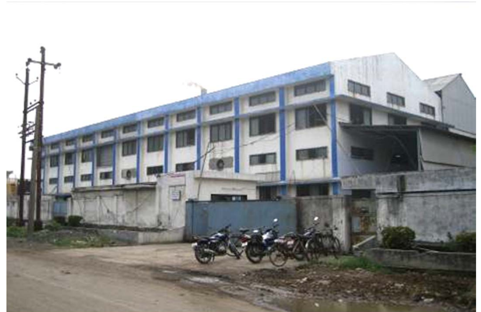
Plant buildings with gates and guard post
