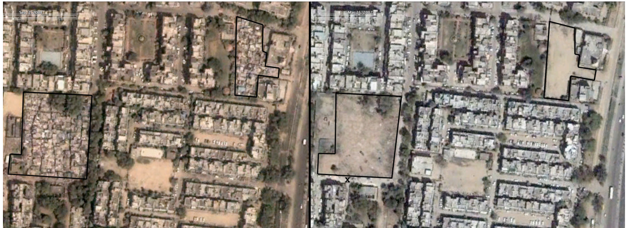
Figure 12. The left and right photographs show two settlements, outlined in black, before and after, respectively, the DDA demolished them on May 4, 2006. The larger of the two settlements, located on the left side of each of the two photographs, is the site of Sant Ravi Das Camp, and the smaller settlement located on the right side of the photographs is what was known as Sanjay Camp. Both photographs were captured from Google Earth and are satellite photographs taken in September 2004 and September 2006, respectively. The small “x” on the photograph on the right (shown below the former site of Ravi Das Camp) shows the position from which the photograph shown in Figure 13 was taken. © Google 2009.
