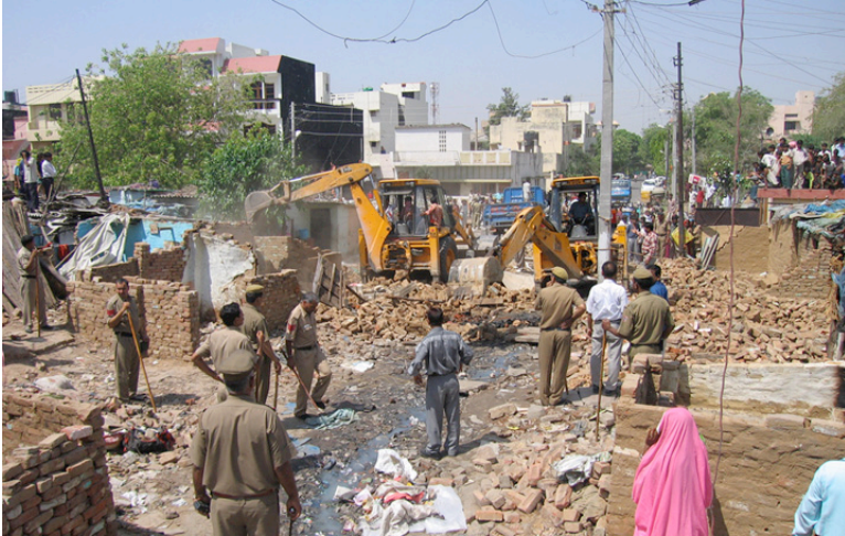
Figure 29. Demolition of 122 jhuggis in Shiv Camp, April 19, 2007. Photo by author.
