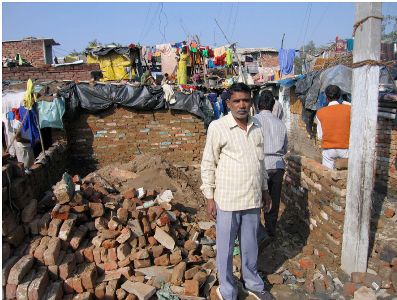
Figure 17. Rebuilding a Shiv Camp hut. Photo by author.
