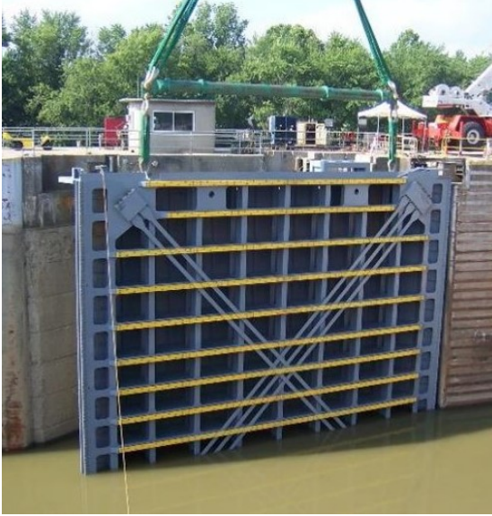
Fig. 1: An open miter gate.
