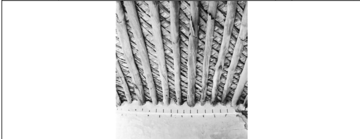
Figure 17. The bayt 'araby roof consisted of large shandal or mangrove beams that supported a layer of woven bamboo columns or basjeel which was then overlaid with woven sheets of reed from Iraq called al-Barria , that was topped with an eighteen inch thick layer of mud and straw. (Source: Lautrette)
