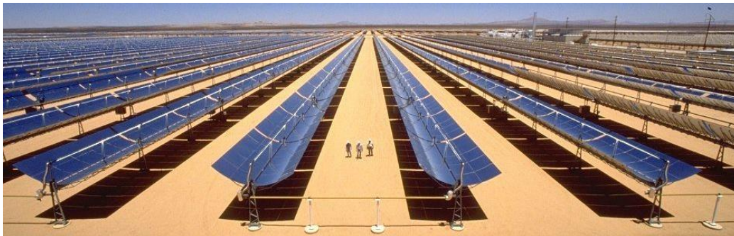
Figure 1.1 – Solar Electric Generating Systems (SEGS) Plant
