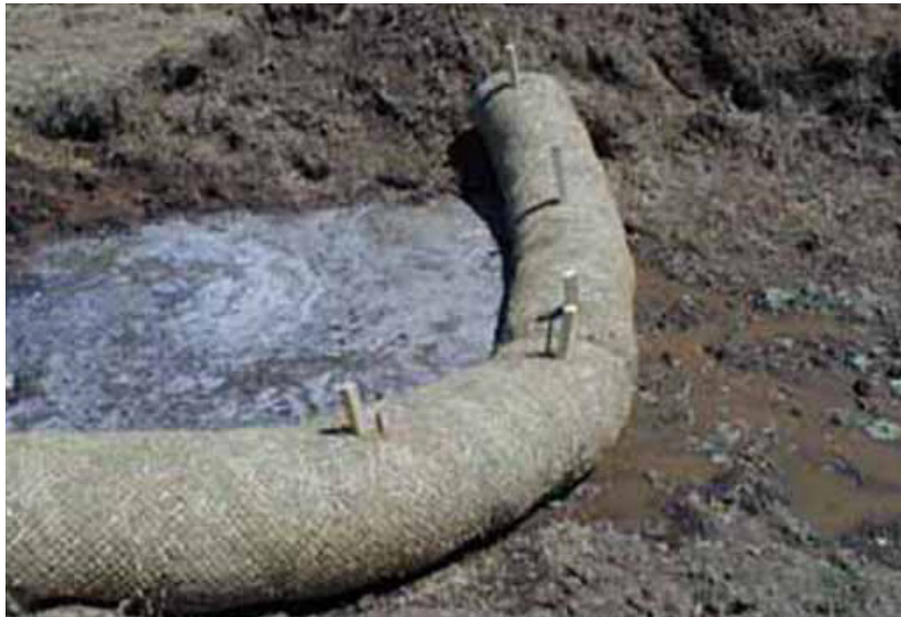
Figure 11. Straw wattles for erosion control. Photo: L. Schwankl
