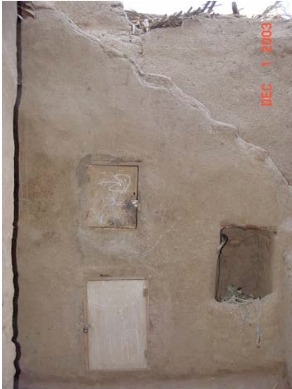
Figure 37. House Three: Cupboards are built into the space beneath the solid staircase (photograph by author).
