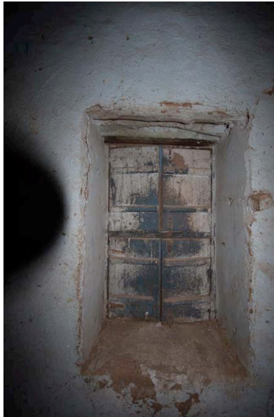
Figure 15. House Two, top and bottom: master bedroom: Windows with four-leafed wooden shutters (photographs by author).
