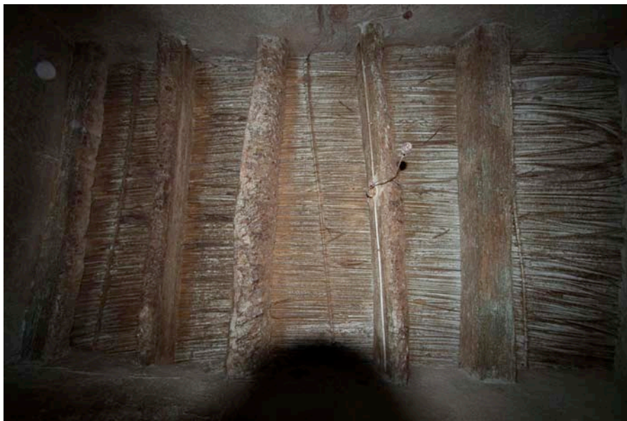
Figure 17. House Two: Roofing made of halved palm trunks and reed matting, plastered and whitewashed (photograph by author).
