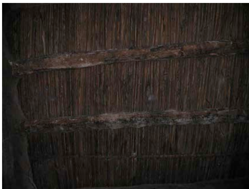
Figure 5. House One Bedroom: Wattle-and-daub roofing (view from beneath) (photograph by author).
