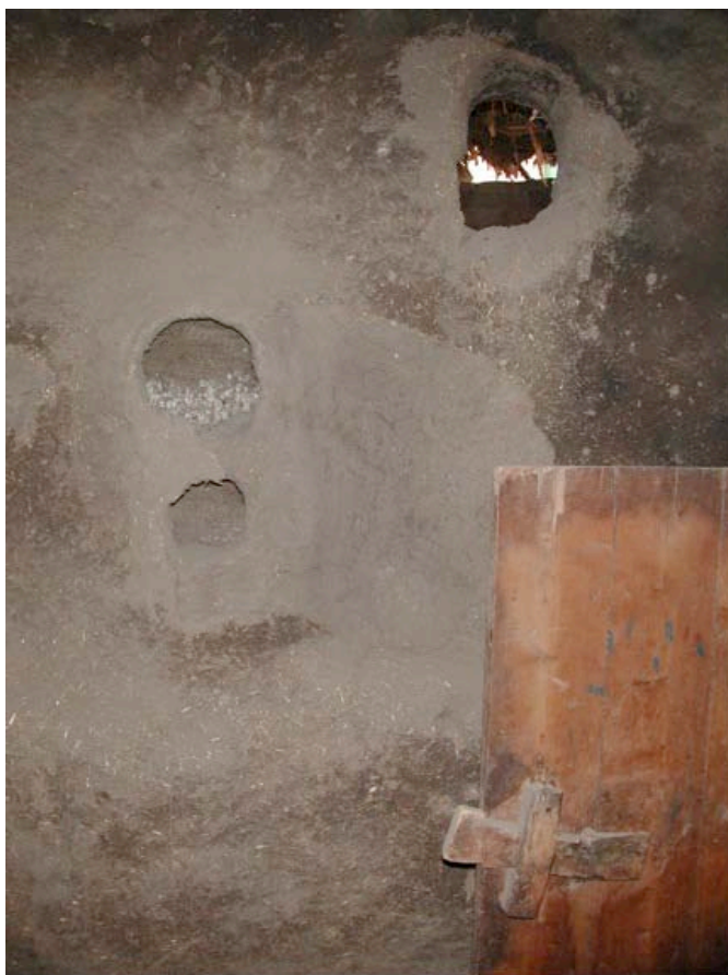
Figure 4. House One Bedroom: door with traditional lock; in wall at left, secret compartments opened up; at upper right, opening in wall for ventilation (photograph by author).
