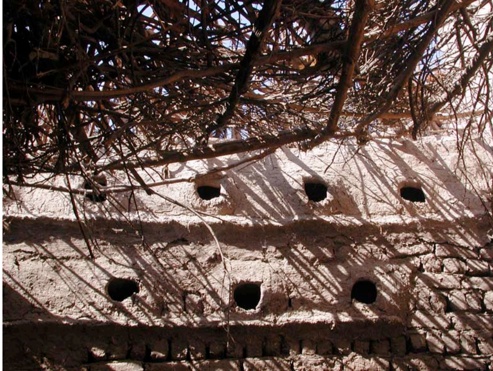
Figure 29. House Two: Horizontally arranged dovecote in courtyard (photograph by author).
