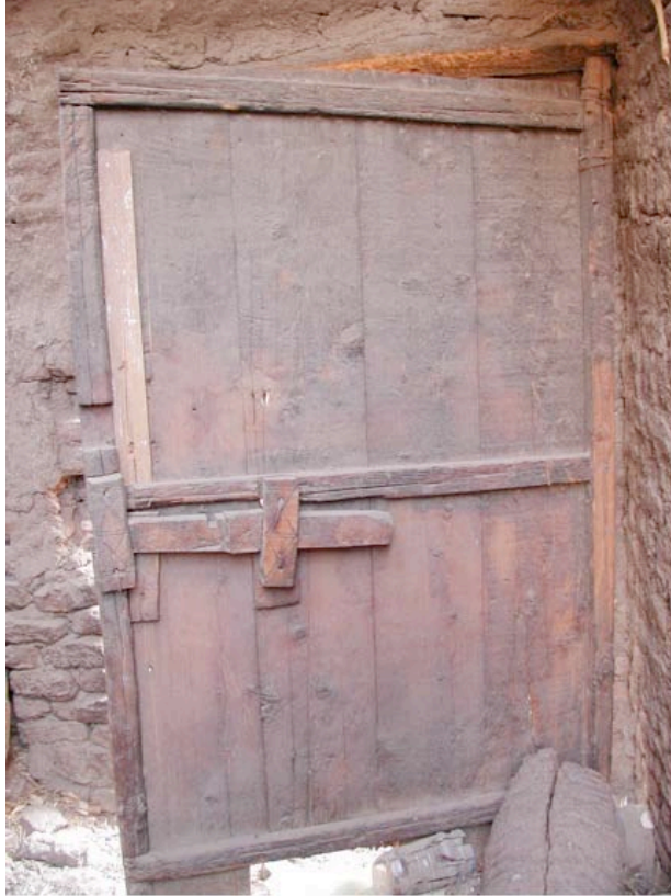
Figure 2. House One: Entrance door with pivot socket and original lock and key (photograph by author).
