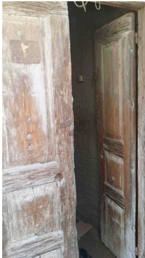
Figure 52. House Four: Western-influenced double-leafed door on metal hinges, with metal bolt (photograph by author).
