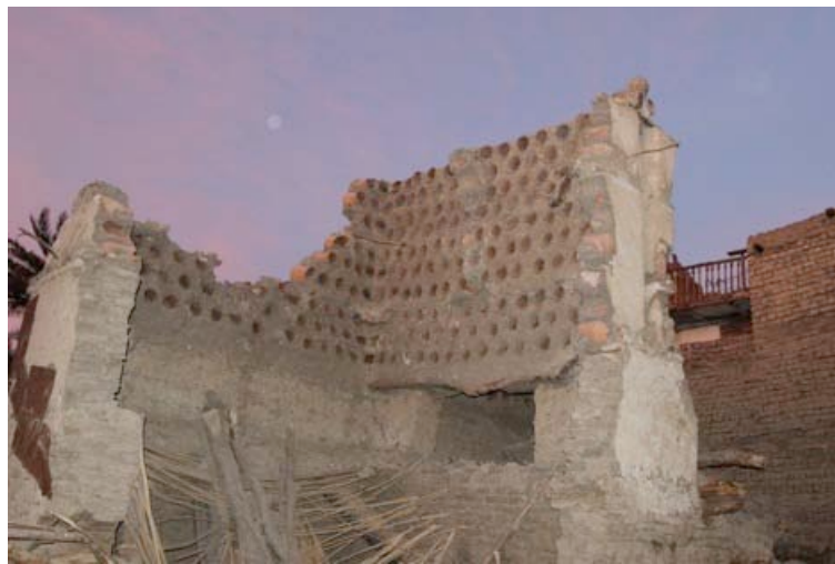
Figure 8. House One: Tall dovecote with embedded pottery vessels vertically aligned (photograph by author).
