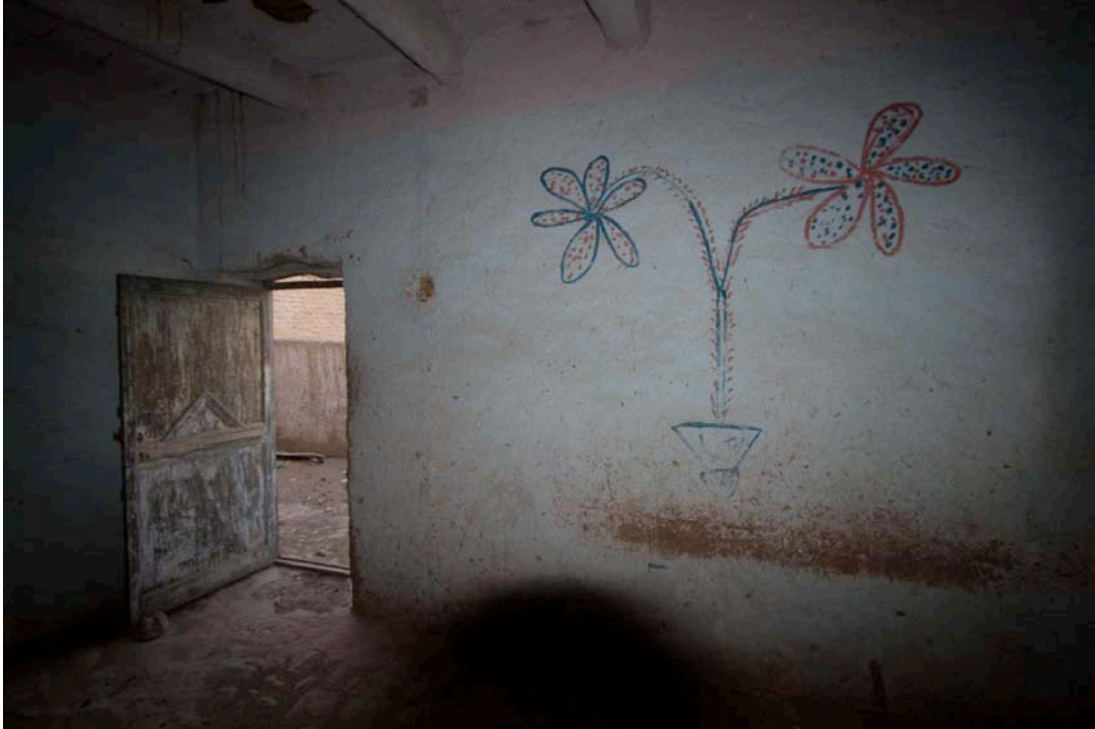
Figure 18. House Two: Master bedroom: Walls painted with floral motifs; flooring is of plastered mudbrick (photograph by author).
