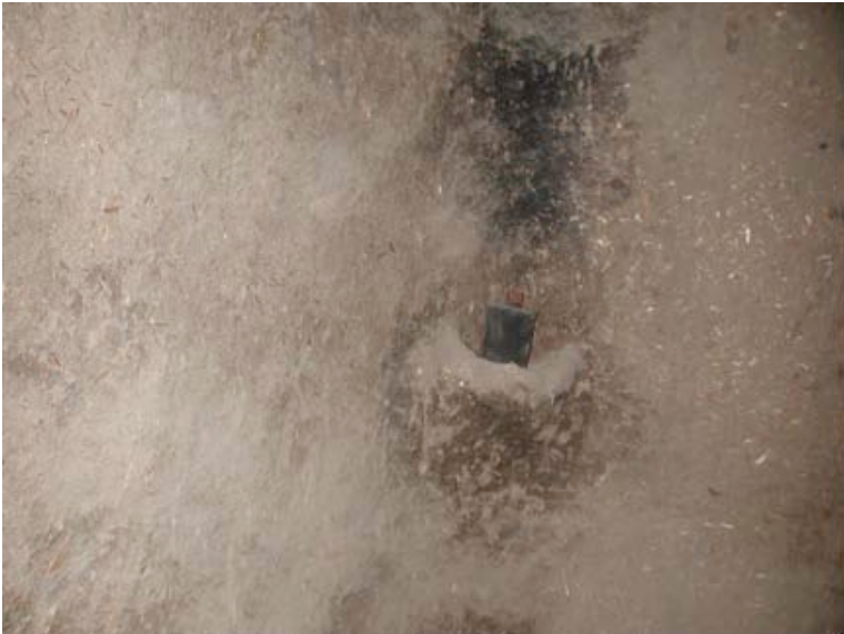
Figure 7. House One Bedroom: Small mud shelf supports kerosene lamp (photograph by author).
