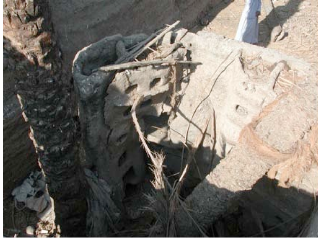
Figure 8. House One: Tall dovecote with embedded pottery vessels vertically aligned (photograph by author).
