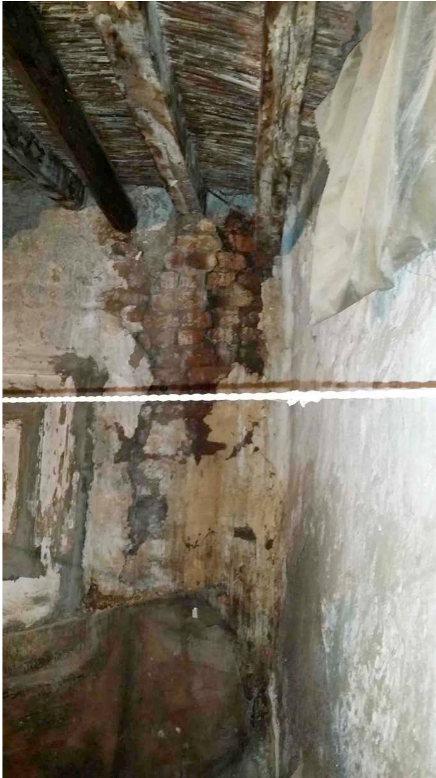
Figure 51. House Four: The roof of western 4" x 4" beams overlaid with palm-rib matting, mud-plastered on top and white-washed on the underside (photograph by author).
