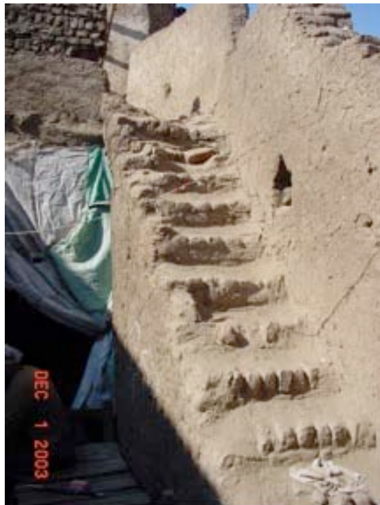
Figure 41. House Three: In open court, mudbrick staircase to roof and pigeon room. Utilitarian tarps hang at left (photograph by author).
