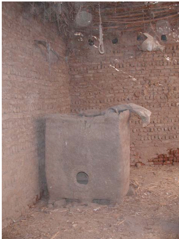
Figure 30. House Two: A şafağ in courtyard; the top has completely broken off (photograph by author).
