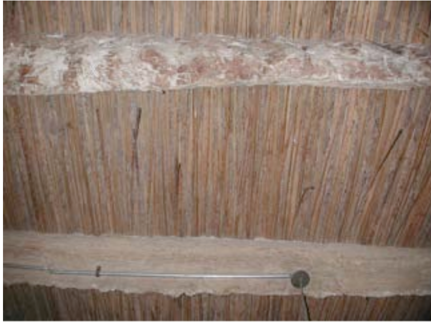
Figure 32. House Three: Roofing of split palm trunks, palm ribs, and reeds, plastered with mud (photograph by author).
