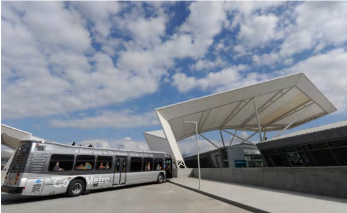
Transit Center - El Monte , Regional bus facility incorporating Off Street bus layover zone, energy-producing photovoltaic panels, use of natural, local resources and materials, and exemplary storm water management system.
