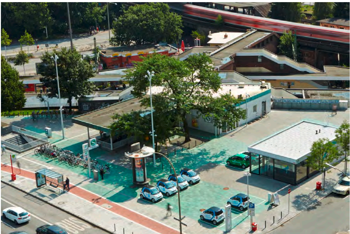
Figure 22. HVV Switch Station (Hamburg)
