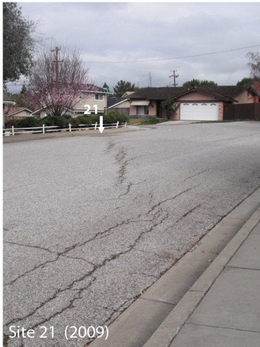
Figure 3.13: Field photos of en echelon cracks at sites 10–13 and 21–23. Both sites have been repaved since these photos were taken.
