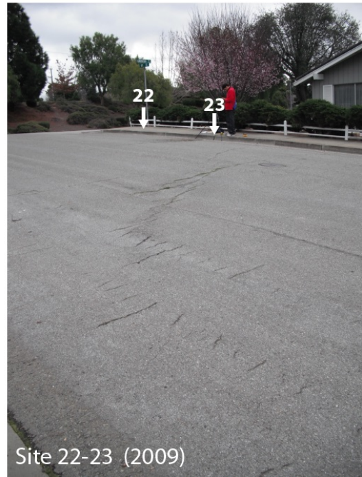
Figure 3.13: Field photos of en echelon cracks at sites 10–13 and 21–23. Both sites have been repaved since these photos were taken.
