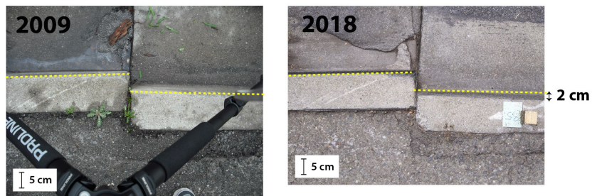
Figure 3.18: Comparing 2009 photos to 2018 photos that show visual differences in the curb perpendicular offset (i.e., sites 12, 24, 35) and in the curb parallel opening (i.e., sites 12, 23, 24). The yellow dashed lines align with the 2009 photos which are overlain on top of the 2018 photos and the difference is shown on the margins.
