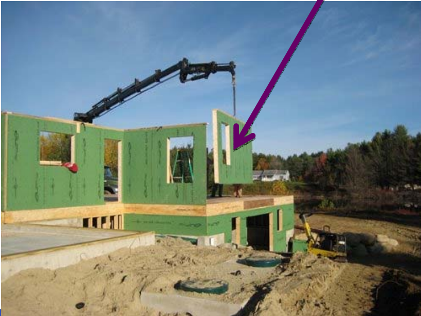
Prefabricated walls
