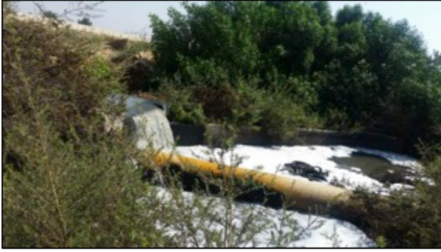
Figure 18. Sewage flows between the mangroves of the coast of the Jazan region.
