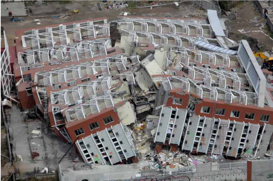
Fig. 1 - Alto Rio building after the earthquake (from http://skyscraperpage.com/cities/?buildingID=85186 )
