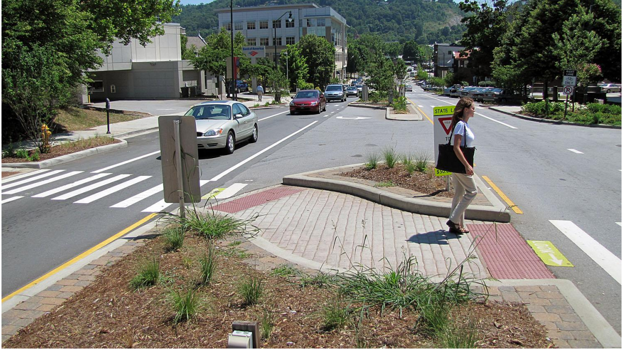
FIGURE 27: RAISED MEDIAN WITH PEDESTRIAN REFUGE
