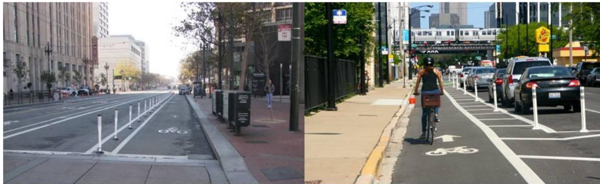
FIGURE 26: CYCLE TRACK EXAMPLES. (L) BOLLARDS FROM SAN FRANCISCO (R) PARKING PROTECTION AND BOLLARDS, CHICAGO
