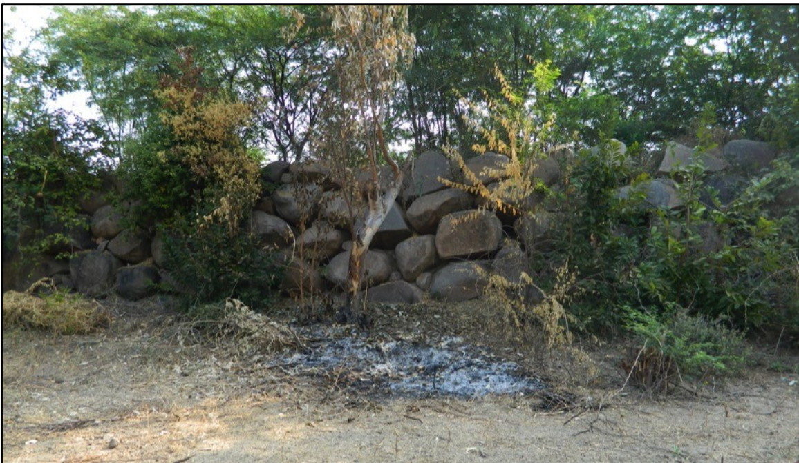
Fig. 6-3: Maliabad outer fortification wall, facing South-West. The height of the wall here is about two and a half meters and the boulders are more or less piled on top of each other without being worked into a geometric shape.
