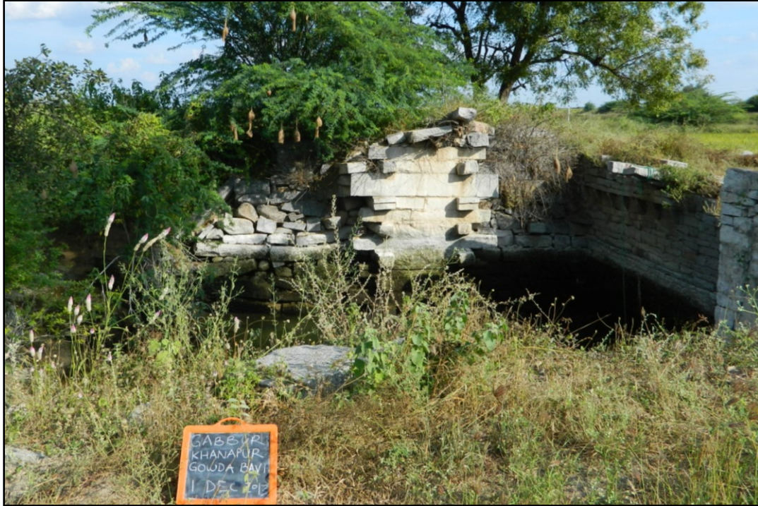
Fig. 5-25: Well (G90) just North of Khane Kere with evidence of repair over time and two styles of masonry.
