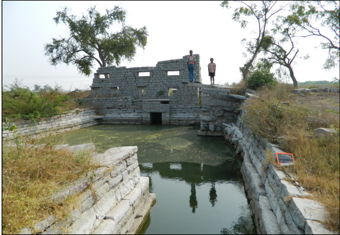
Fig. 5-27: Ragam Bavi (G131) with a sluice opening and the older water lifting area (where the two boys stand).
