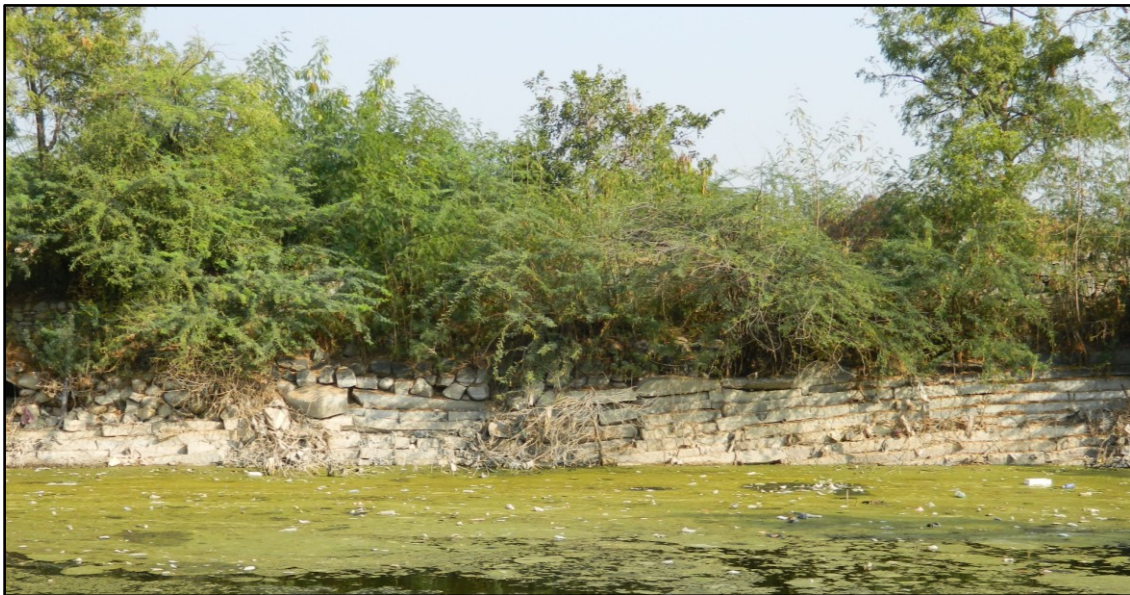
Fig. 5-11: Sakkar Bavi (G28) masonry along eastern edge.
