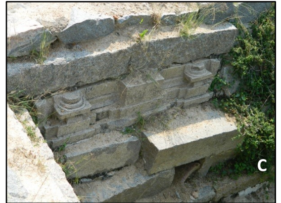
Fig. 8-1: Structural reuse in embankment masonry. Remains of a pilaster (A) and a panel of elephants (B), reused to construct the embankment of reservoir R1 at Maliabad. Part of a wall-shrine (C) reused in masonry of an outlet from reservoir R2 at Maliabad.
