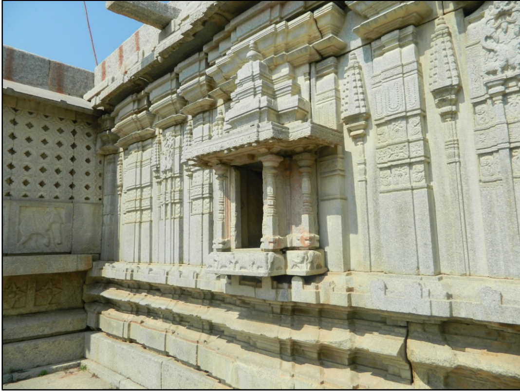
Fig. 5-51: Venkatesvara temple, wall-shrine enclosing a niche, aedicular components, and double nasi on a staggered wall-shrine projection, around the eastern shrine.
