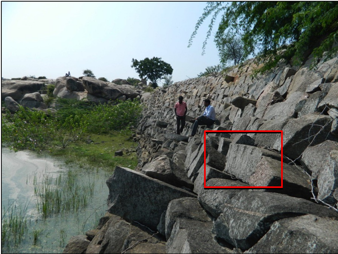
Fig. 6-21 Masonry of R2 embankment and quarry marks on its stone blocks.
