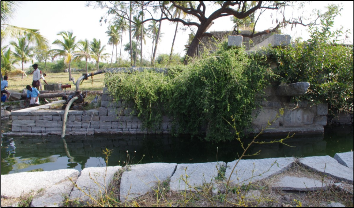
Fig. 5-37: Well (G63), water lifting area connected to a channel/narrow canal for field irrigation. A few naga stones and a Nandi sculpture were also found next to this well.
