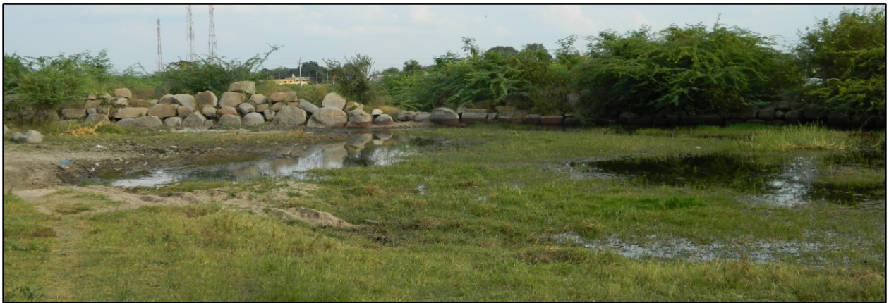
Fig. 5-45: A bund constructed out of boulders, south-west of Gabbur and south of the Suguresvara hill.
