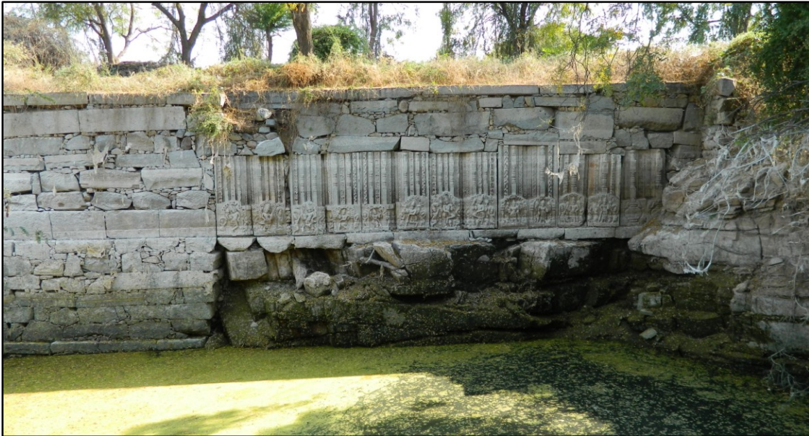
Fig. 5-6: Well at G83, looking south, about seven pairs of door-jambs arranged to form the masonry. Every year after the monsoons the well fills up enough to submerge the door-jambs.
