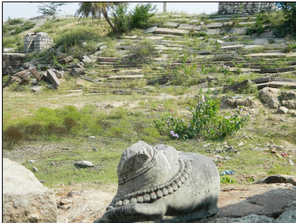
Fig. 5-13: Devanapalli embankment masonry from inside the dry reservoir; damaged Nandi bull image on a rocky outcrop in the foreground.
