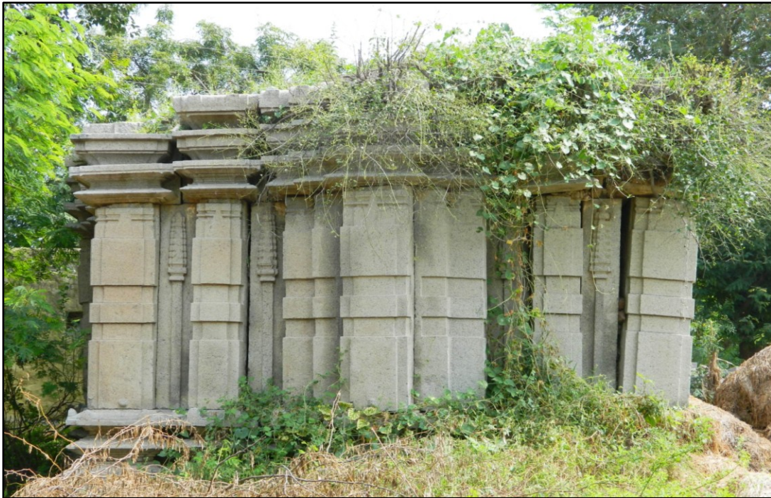
Fig. 5-52: Staggered square plan of the shrine at Hampayyana temple, with kuta stambha as the aedicular component.
