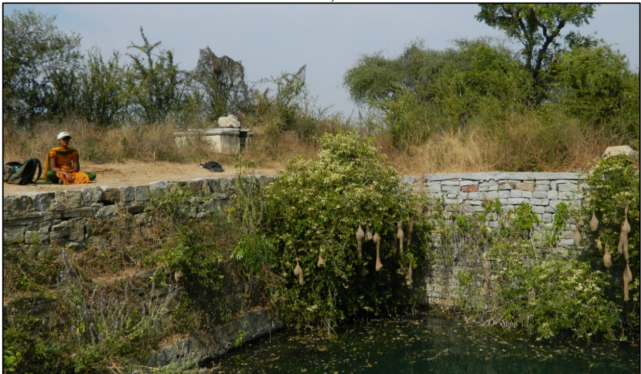
Fig. 5-28: Basavanna Bavi (G98), along the embankment of Basavanna Kere, with stone masonry
