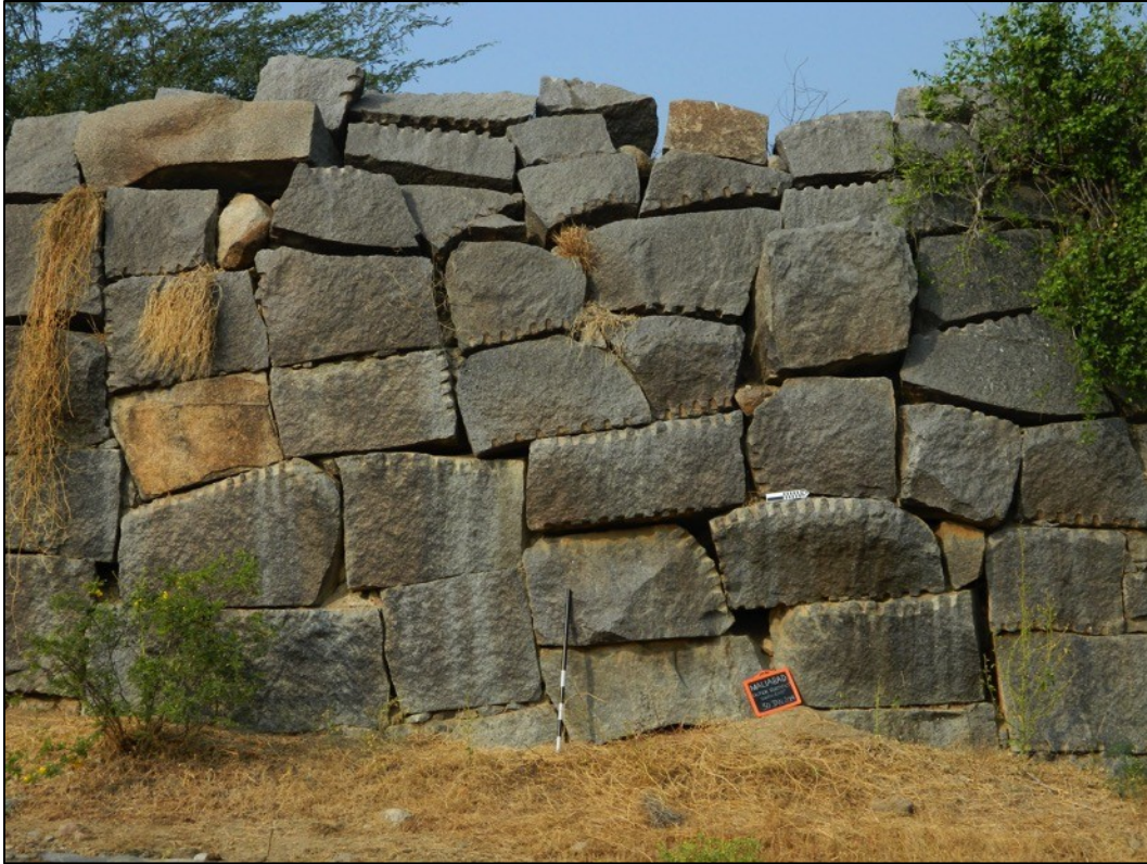
Fig. 6-2: Maliabad outer fortification wall, facing East.
