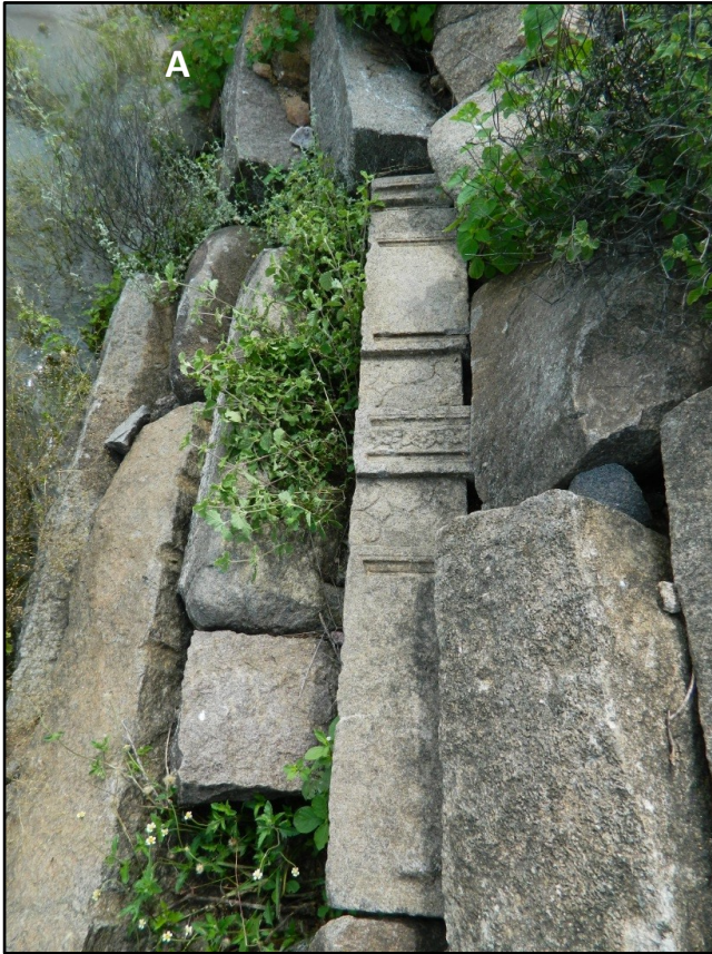
Fig. 8-1: Structural reuse in embankment masonry. Remains of a pilaster (A) and a panel of elephants (B), reused to construct the embankment of reservoir R1 at Maliabad. Part of a wall-shrine (C) reused in masonry of an outlet from reservoir R2 at Maliabad.
