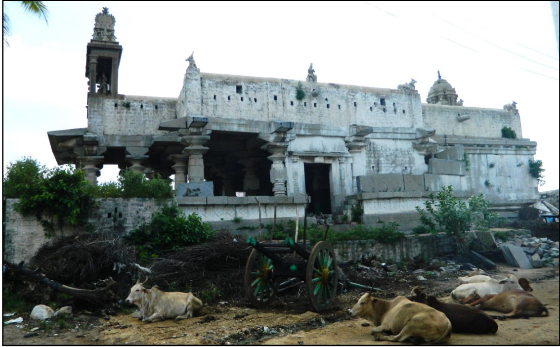
Fig. 5-49: Mel Sankara temple (G28), western side. Note the modern constructions (e.g., the parapet) are incorporated into the medieval architecture. Plain slabs of stone are used in constructing the vimāna , which is of a square plan.
