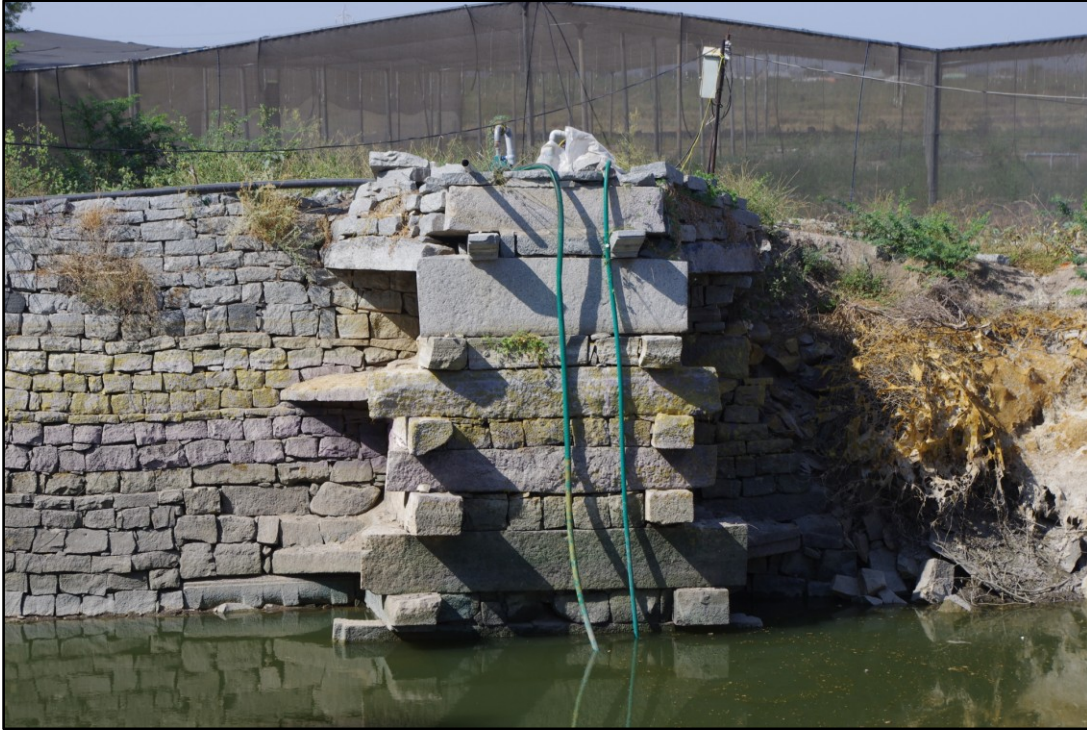
Fig. 5-41: Well (G124) and water lifting area next to a small embankment. A naga stone was found close to this well on the embankment. Older structural remains can be seen incorporated into the new well masonry.
