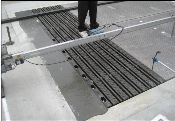
Figure 3.4: Laser profilometer recording surface profile of the Trelleborg unit.
