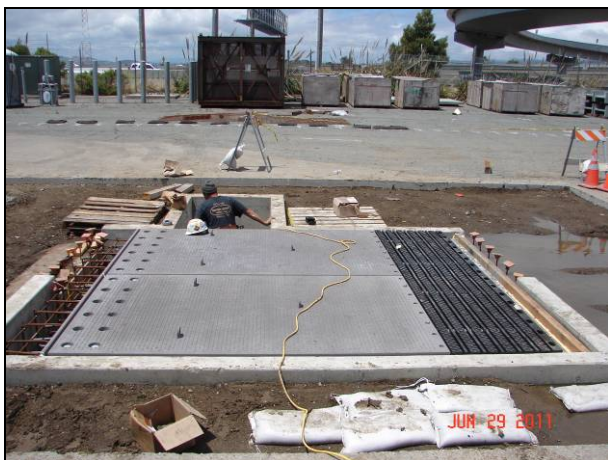
Figure 2.8: Completed steel plate installation.
