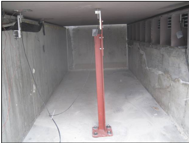
Figure 3.10: General view of instruments underneath steel plate.
