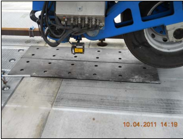
Figure 4.41: Phase 3.1: Impact load from neoprene step.
