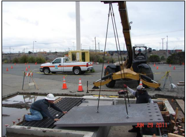
Figure 2.7: Steel plate installation.
