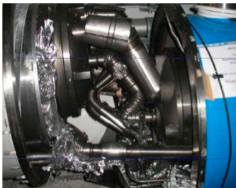
Figure 1: A severely damaged interconnect.
