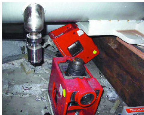
Figure 2: A broken magnet support.
