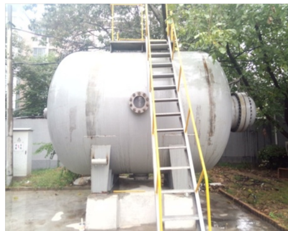
(b) the pressure tank for implosion test
