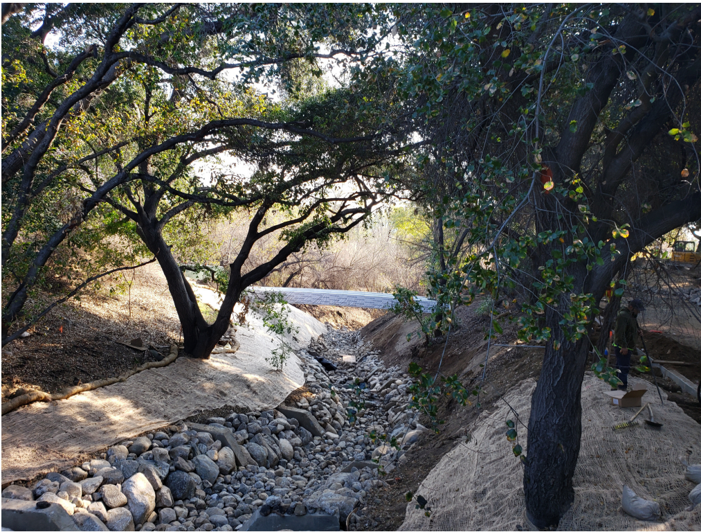
Figure 11 : The Berkshire Creek restoration project completed in Los Angeles County
