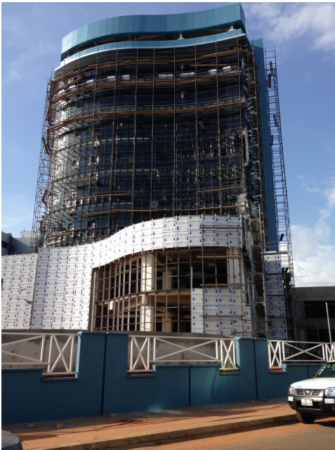
Figure 3: Construction in progress
