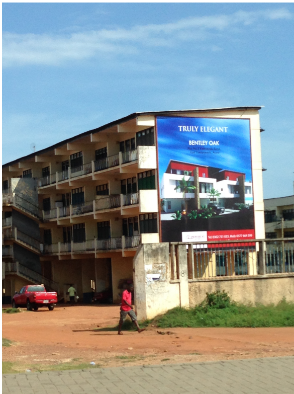
Figure 11: Deteriorating government-built apartment block for the presidential guard during the Nkrumah era provides advertising space for “Bentley Oak,” a new luxury condominium development
