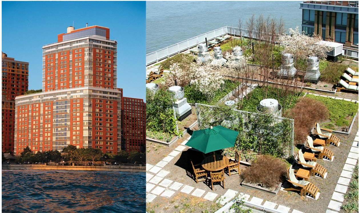
Figure 2.5: The Solaire building in New York, New York, USA (left) which is a residential apartment building that reclaims building wastewater for toilet flushing and cooling systems and reclaims stormwater for irrigation of a rooftop garden (right) (Consentini (2022)).
