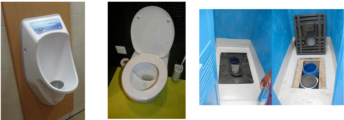
Figure 1.3. Urine-diverting toilets. From left to right: waterless urinal, NoMix flush toilet, urine-diverting dry toilet.
