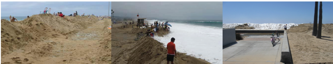
Figure 1.1: Temporary sand berm constructed at Newport Beach in 2010.
