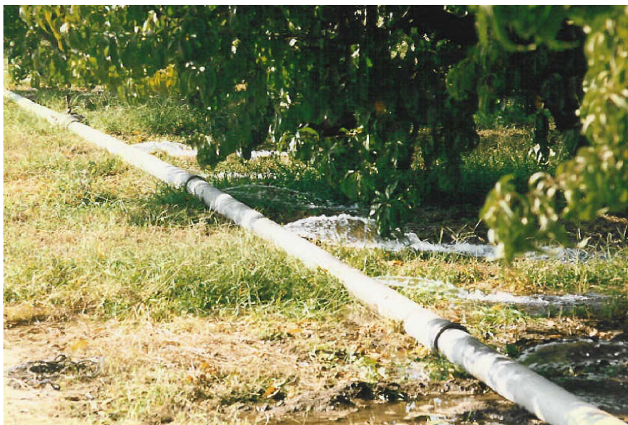
Photo 4. Another view of the irrigation pipe.
