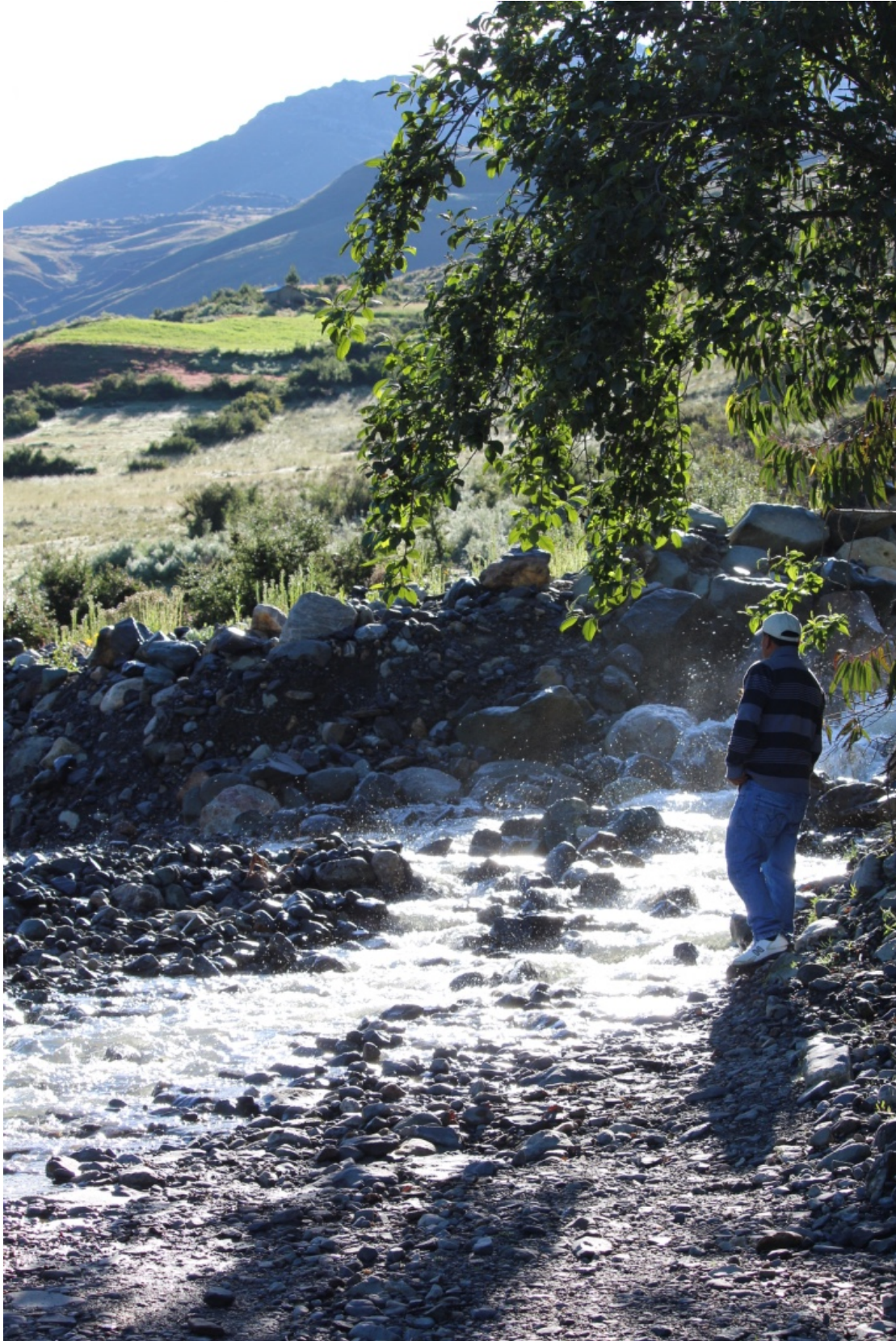
Figure 72 The entire road washed away from the force of the rain, building a new river through the campo
