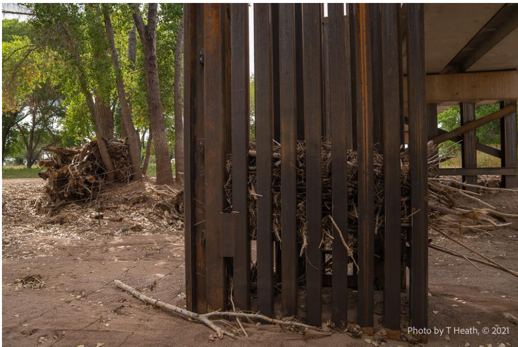
Figure 13: Woody debris accumulation following the August 2021 floods at the San Pedro River border wall. Photo by Tony Heath.
