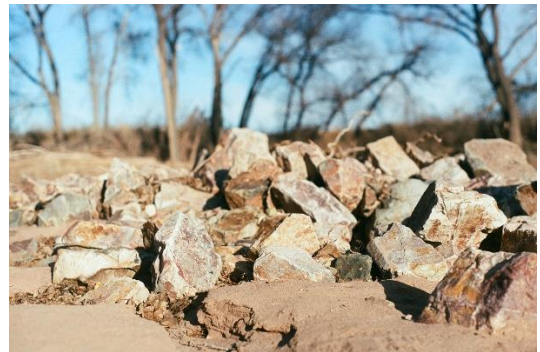
Riprap placed during floodgate construction: large cobbles and small boulders.
