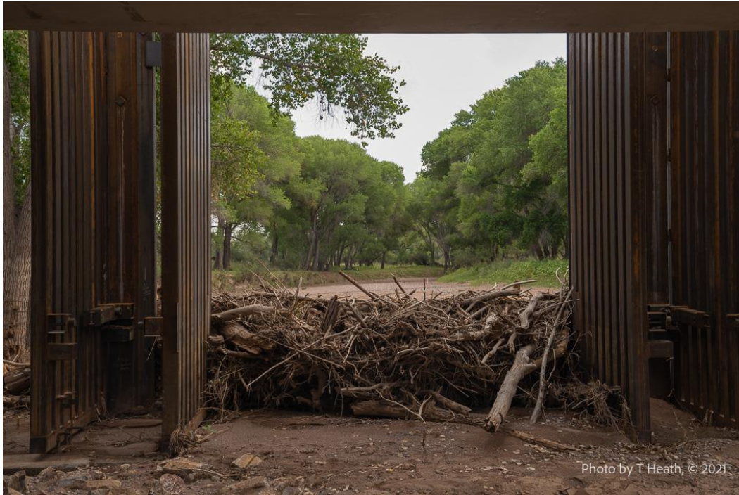
Figure 13: Woody debris accumulation following the August 2021 floods at the San Pedro River border wall. Photo by Tony Heath.
