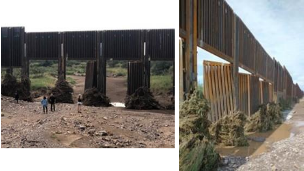
Figure 6: Flood gates torn from their hinges after the August 2021 monsoon on Silver Creek at the US-Mexico border wall. Photos by Fernando Sobrazo / Cuenca Los Ojos.
