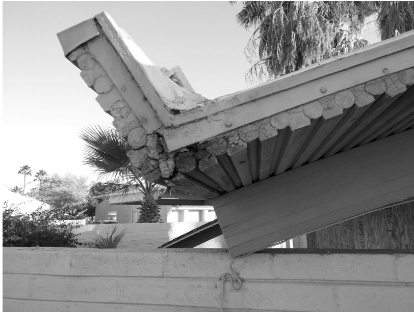
Fig. 6. Detail of the roof construction. (Photograph by Volker M. Welter, 2015.)
