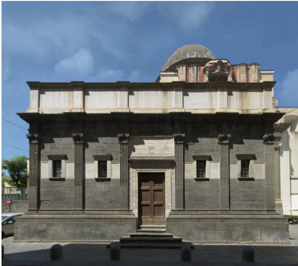
Fig. 2. Pontano Chapel, Naples. View of the façade on Via de' Tribunali.
