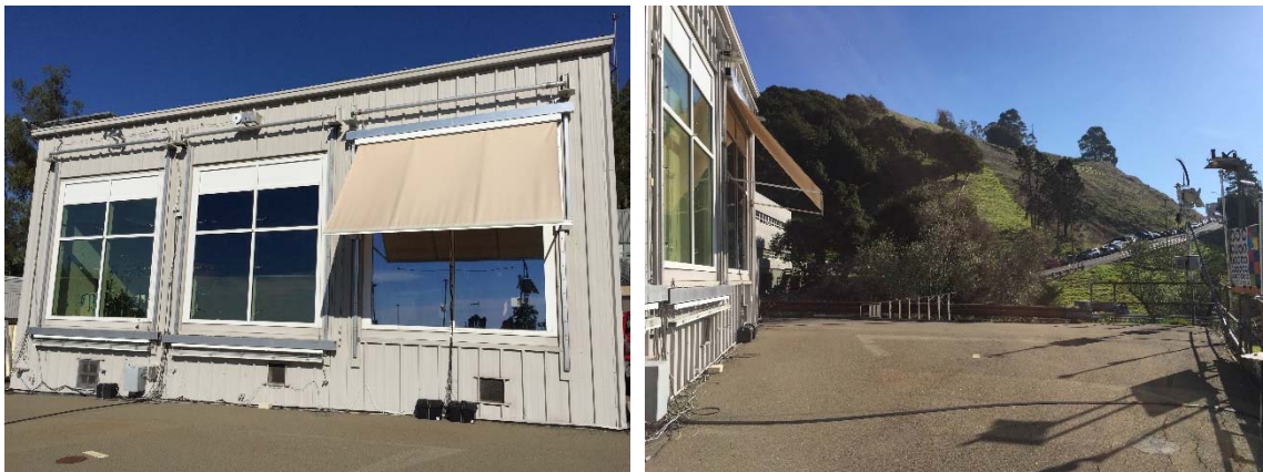
Figure 1. LBL Window Testbeds (71T): (left) exterior and (right) panel installation
