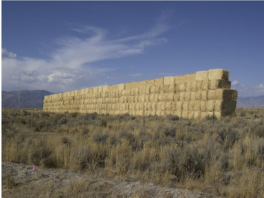
Figure 2.8: Mock straw bale sound barrier, 6 m high and 90 m long. From (Finn et al., 2010)
