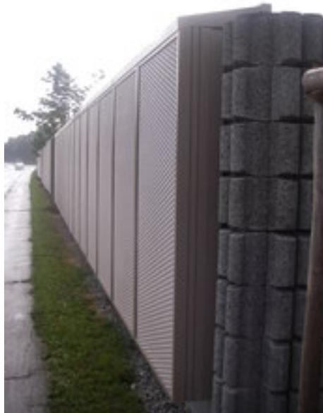
Figure 2.4: Filter panel installed on a noise barrier for the SPAS study. (Magistrat Klagenfurt, 2011)
