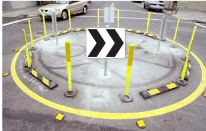
Figure 17. Example of mini traffic circle with bollards suitable for testing (Redondo Beach Public Works, 2016)
