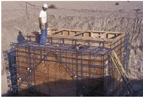
Left and center, construction of the two large weighing lysimeters at KREC began in 1986. Each lysimeter consists of an underground chamber that houses a balance-beam weighing system with a rectangular “flower pot” measuring 6.5 feet wide by 13 feet long by 6.5 feet deep. Right, researchers enter the completed lysimeter.
