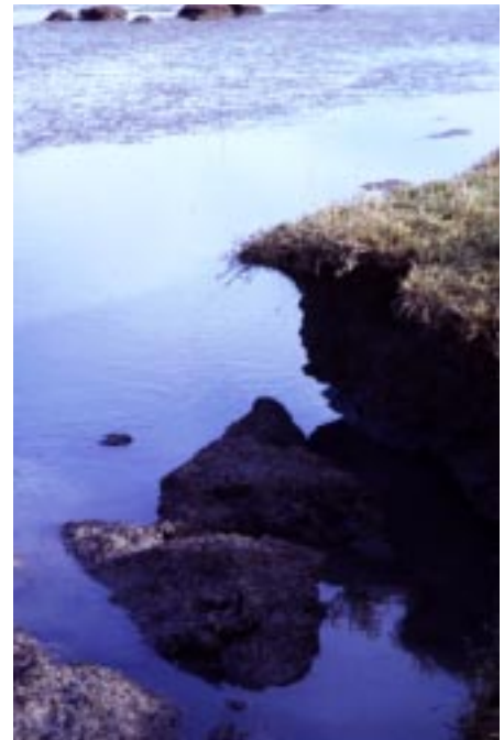
A collapsed marsh bank in San Francisco Bay, caused in part by the presence of burrowing isopods. Photo: Jeff Crooks.
