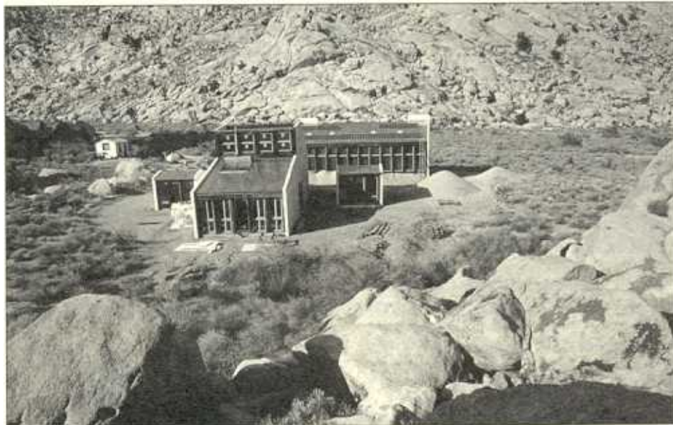
The sun's-eye view of the new passive-solar facility at the Granite Mountains Reserve. In the foreground is the residence building, flanked by two sleeping cabins; behind those is the laboratory.
