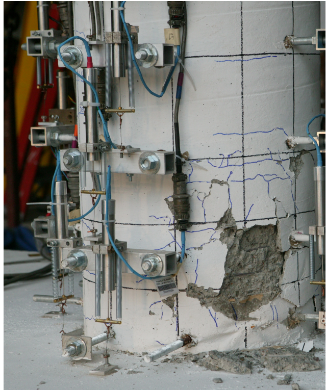
(c) Local spalling of concrete cover and cracking at NW face
