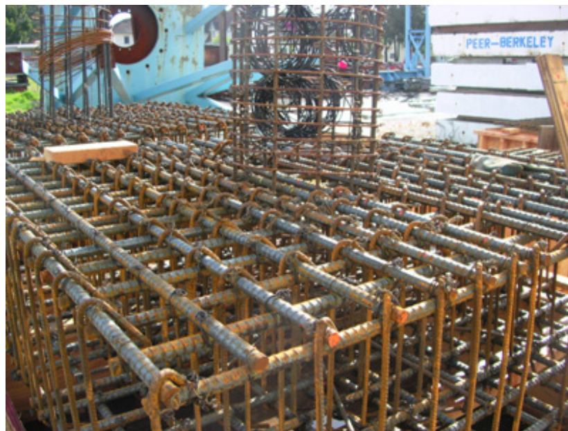
Figure 3-8: Column Cage and Footing Steel
