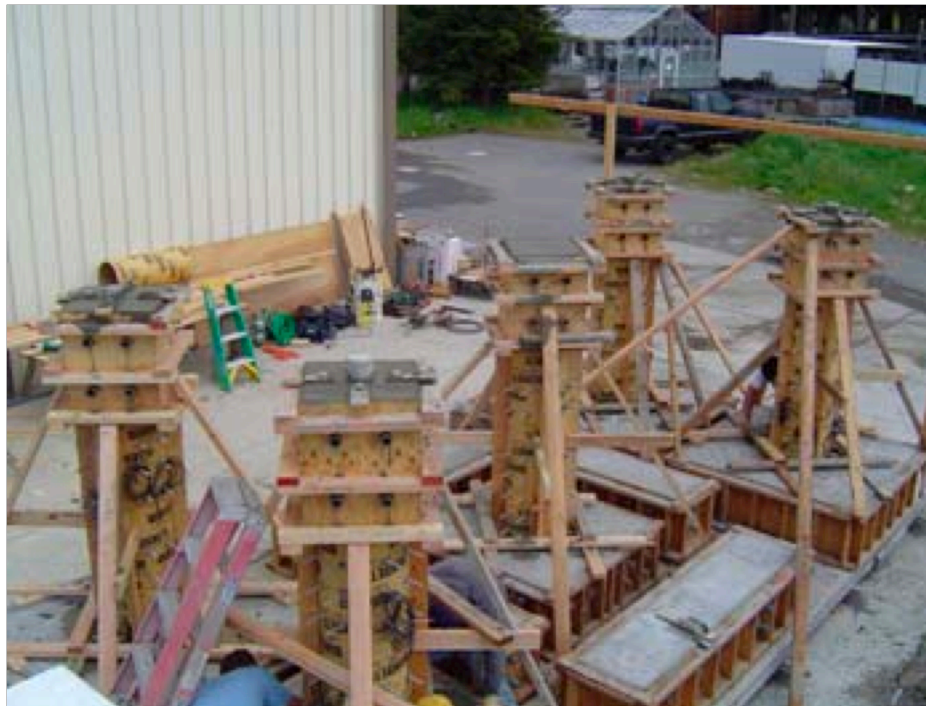
Figure 3-12: Column and Top Block (rocking specimen in center)
