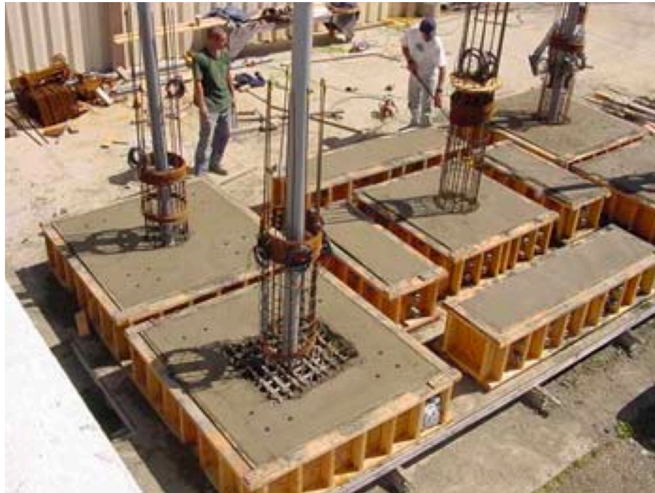
Figure 3-10: Footing and Blocks before column casting (rocking column center of specimens)
