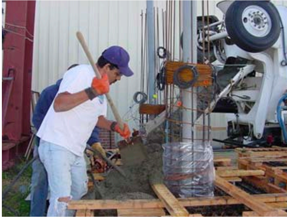
Figure 3-9: Casting footing
