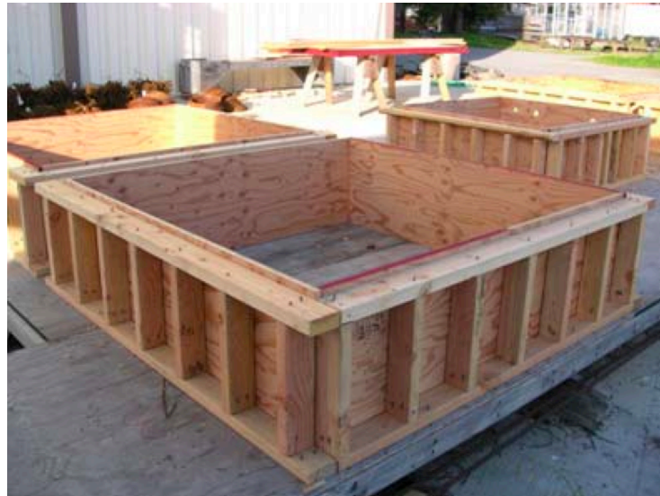
Figure 3-7: Footing Forms (Rocking Column at Top Right)
