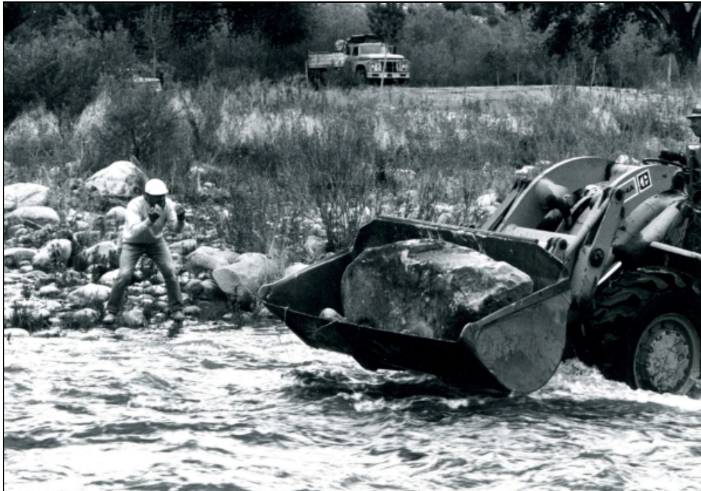
Figure 34. Tom Johnson directs the placement of a large boulder (a) and slalom athletes move a rock into place in the Kernville (b). Photos compliments of Tom Johnson.
