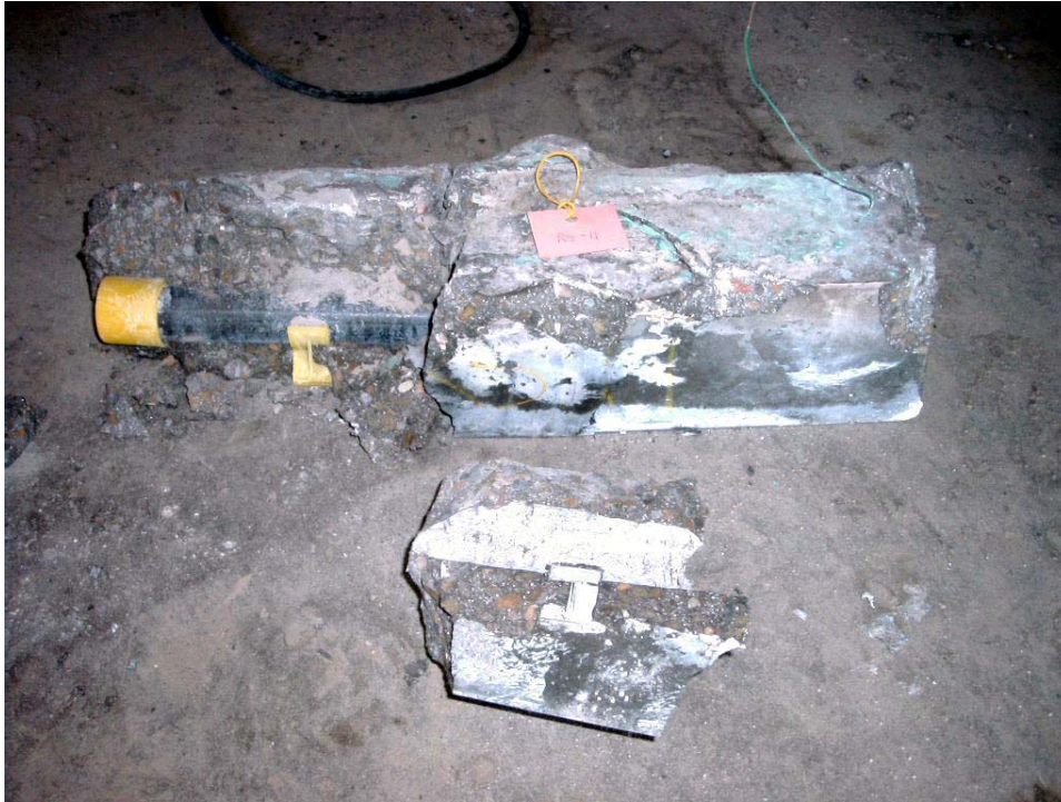
Figure 21. Extraction of dowels for visual inspection.
