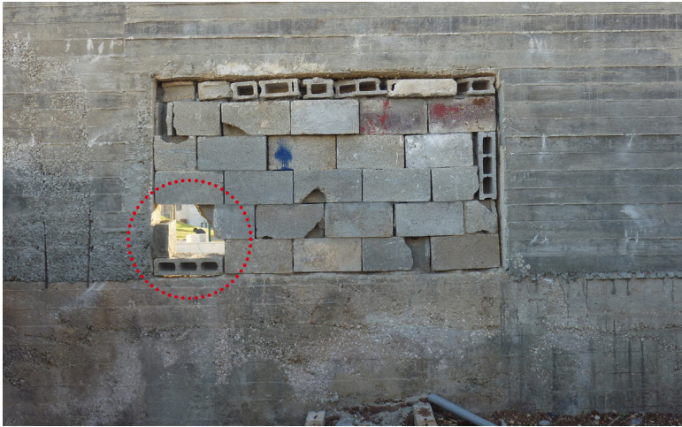
View of the closed window (hole) from Murad's backyard.
