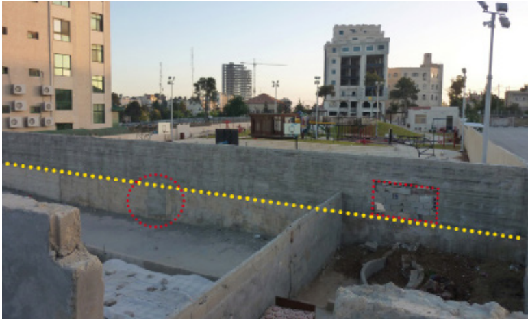
Image of the wall from the refugee camp. Dotted yellow line showing the previous height of wall (below) and the newly added one (above), as well red dotted circle showing traces of former entrance, and window (red dotted rectangle) from behind the wall, (window is from Murad's back yard).
