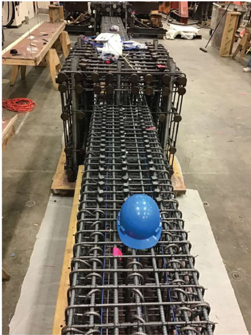
(c) Column cage during construction (top face).
