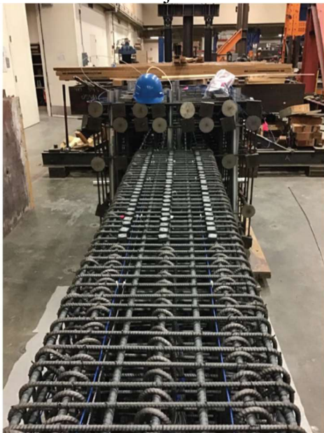
(e) Column Cage during construction.
