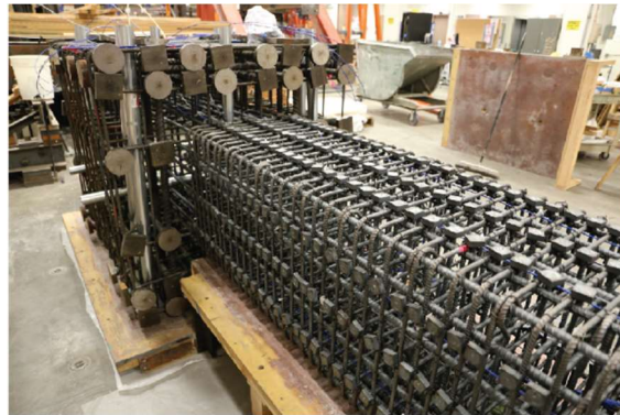
(b) Column cage during construction.
