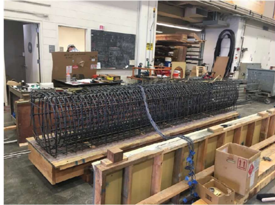
(b) Column cage during construction.
