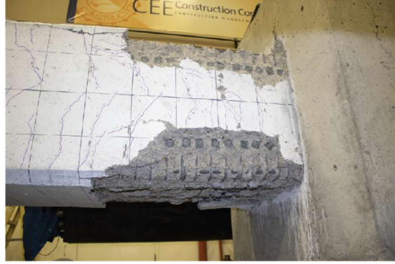
(n) Post-testing column-foundation joint (north side).
