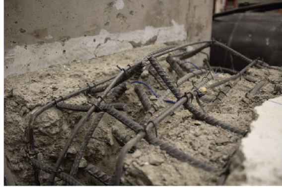
(h) Post-testing column-foundation joint (top face).
