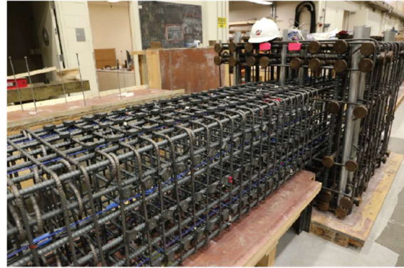
(b) Column cage during construction.
