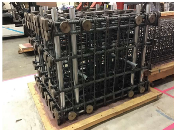
(d) Foundation Block during construction.
