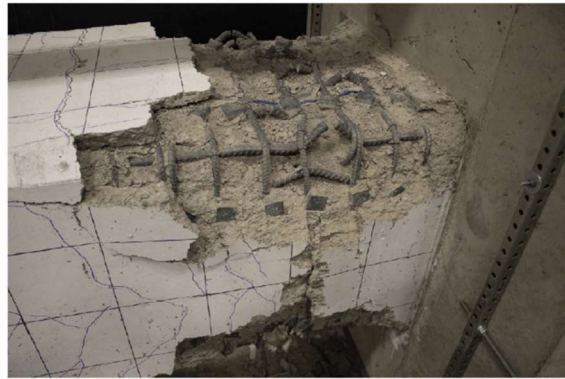
(h) Post-testing column-foundation joint (bottom face).
