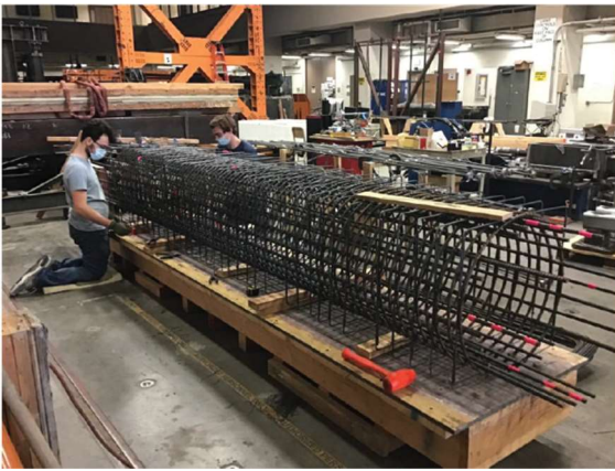
(a) Column cage during construction.
