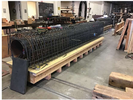
(b) Column cage during construction with steel pipe.
