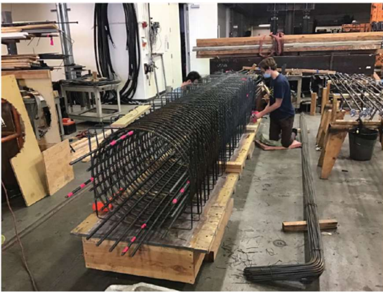
(a) Column cage during construction.
