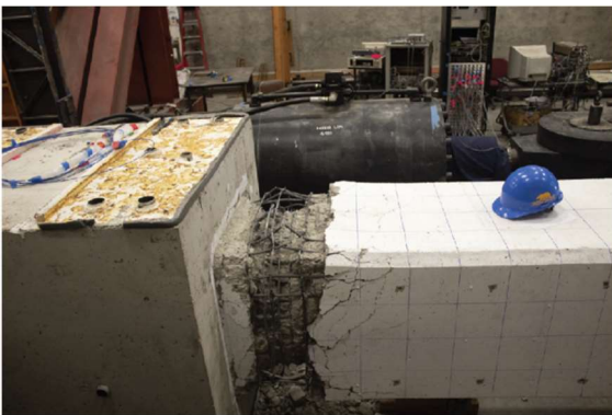
(e) Post-testing column-foundation joint (south side).
