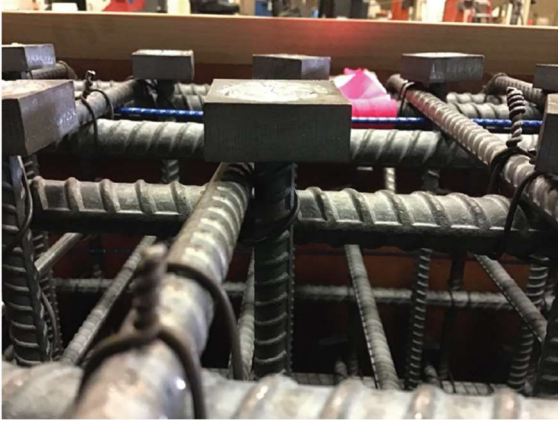
(g) Headed bars placement over hoops.
