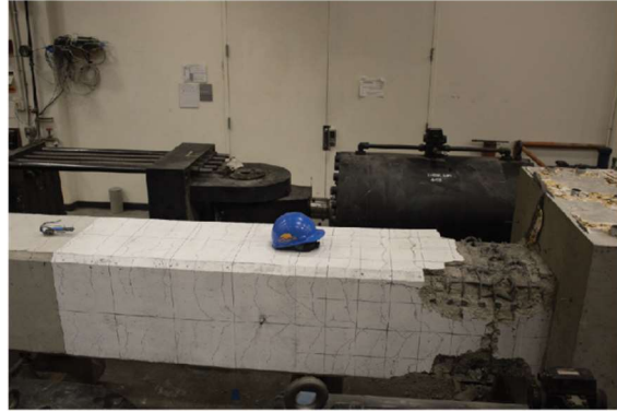
(f) Post-testing column-foundation joint (north side).
