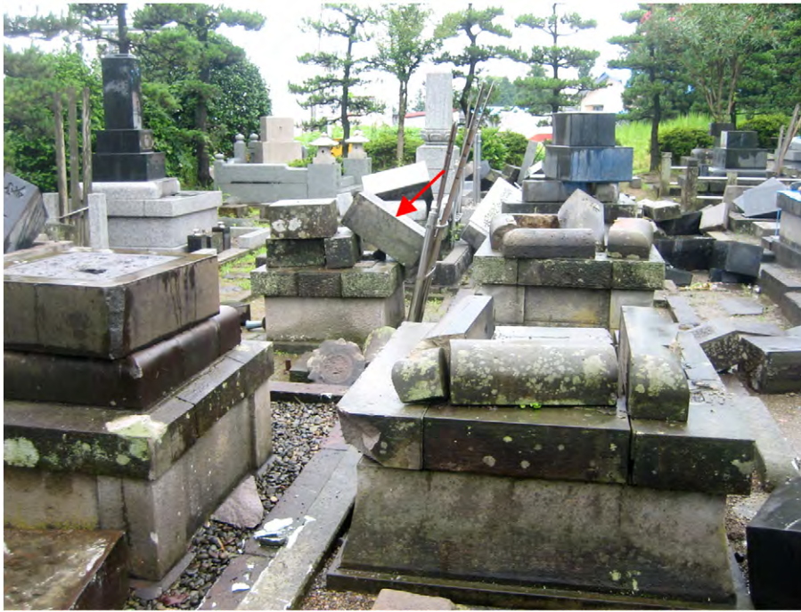
Fig. 4. Toppled monuments at 12 km JMA epicentral distance with approximate 90% topple ratio. Typical width and height of the most slender blocks (arrow) is 25 cm by 75 cm ( b/h = 0.33 ).
