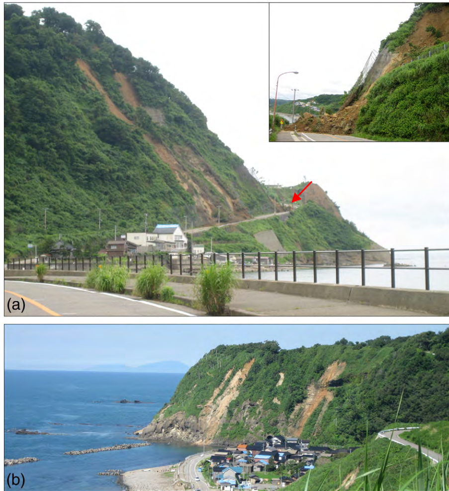
Fig. 2. Coastal landslides (a) north of Kashiwazaki at 3 km JMA epicentral distance and (b) south of Kashiwazaki at 23 km JMA epicentral distance. Arrow in (a) identifies the location of the inset image.
