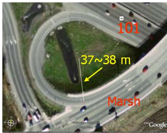
Figure 4.9 On ramp from Marsh Rd. to southbound US 101 (Google map)
