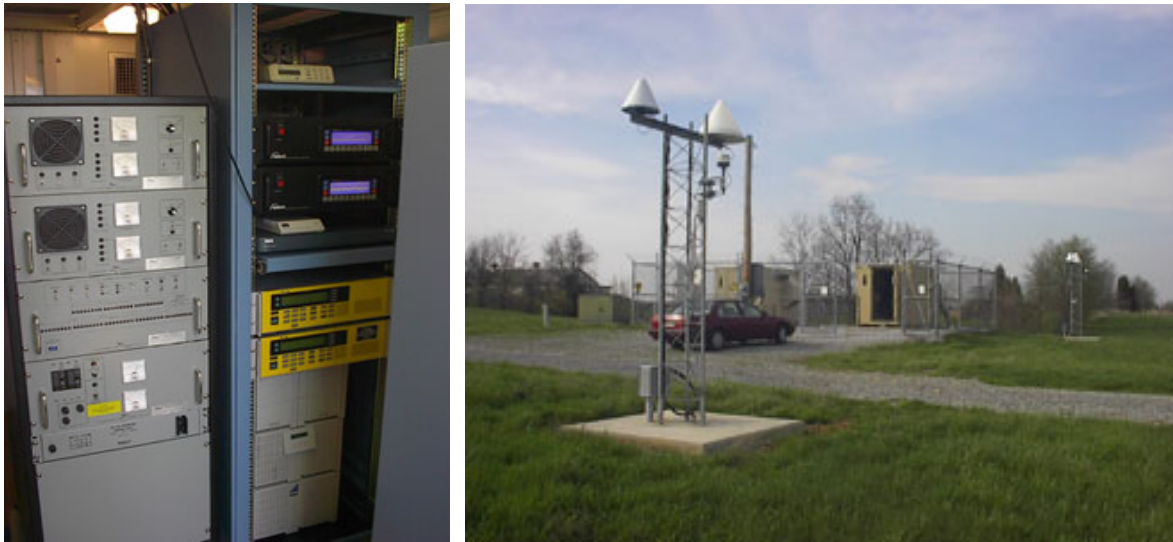
Figure 4.44 Hagerstown, HA-NDGPS broadcast station rack and receiver antennas [FHWA,2002].
