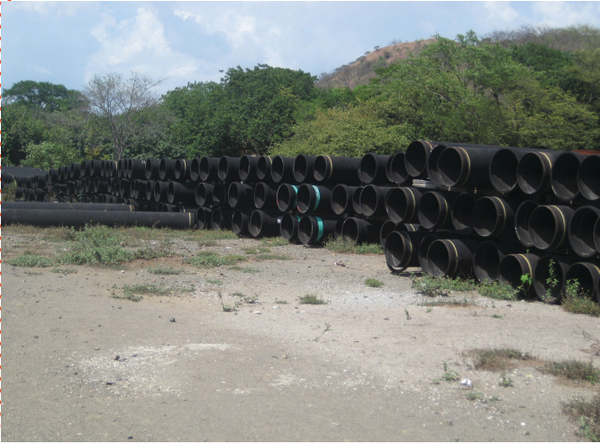
Pipes waiting to be installed near Sardinal. PHOTO: ARCHIVES KIOSKOS SOCIO-AMBIENTALES, UCR COSTA RICA.
