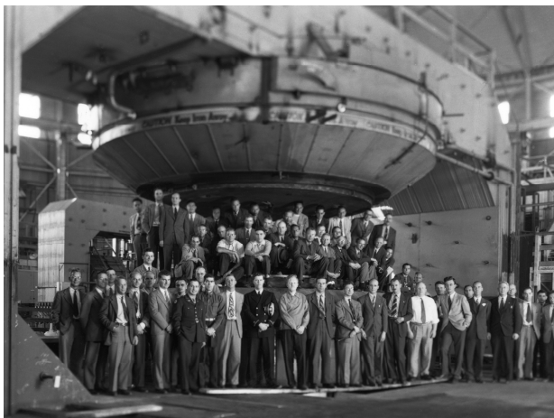
Figure 2. The magnet of the 184-inch cyclotron, the largest that Lawrence built. Courtesy of Lawrence Berkeley National Laboratory.
