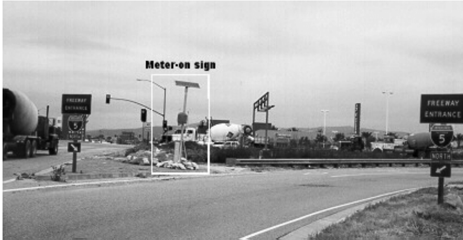
Figure 4-9. Meter-on sign with solar panel at Jamboree Road ramp entrance
