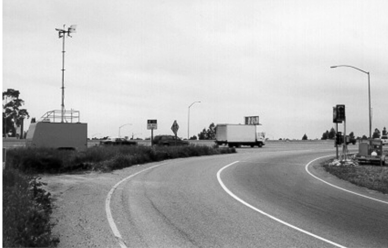
(a) Onramp with surveillance trailer on left, ramp meter trailer and signal on right
