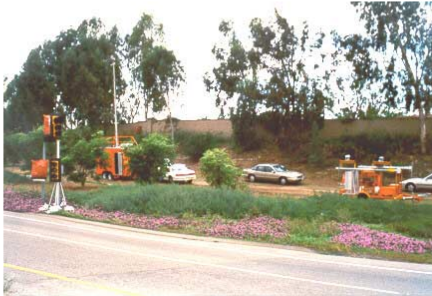
Figure 4-7. Surveillance and ramp meter trailers at Tustin Ranch Road
