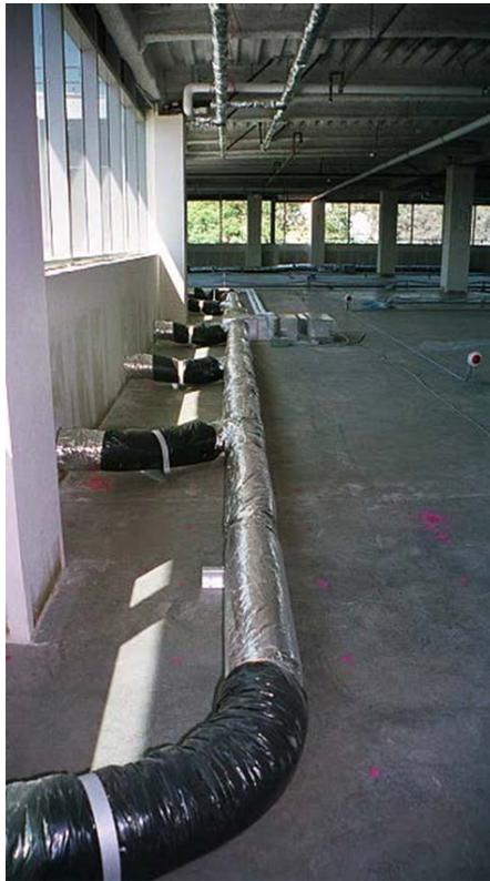
*Figure 3-13. Perimeter fan-coil unit connected to window sill diffusers*
