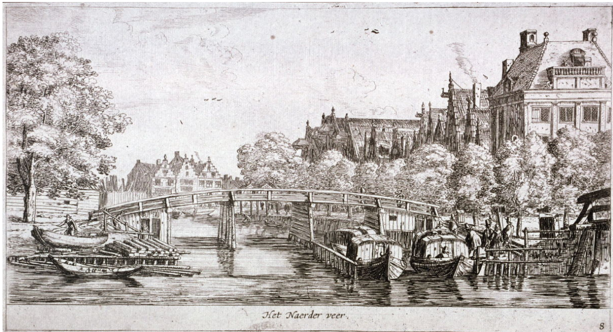
Figure 3.16: Reinier Nooms, The Ferry to Naarden, on the river Amstel , ca. 1659-1662
