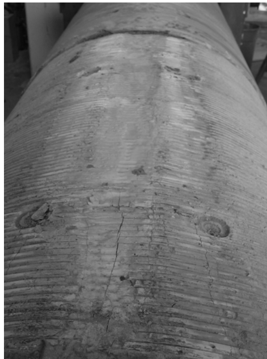
Fig. 25. Concrete core at north side of the splice (see Figures 2 and 4)
