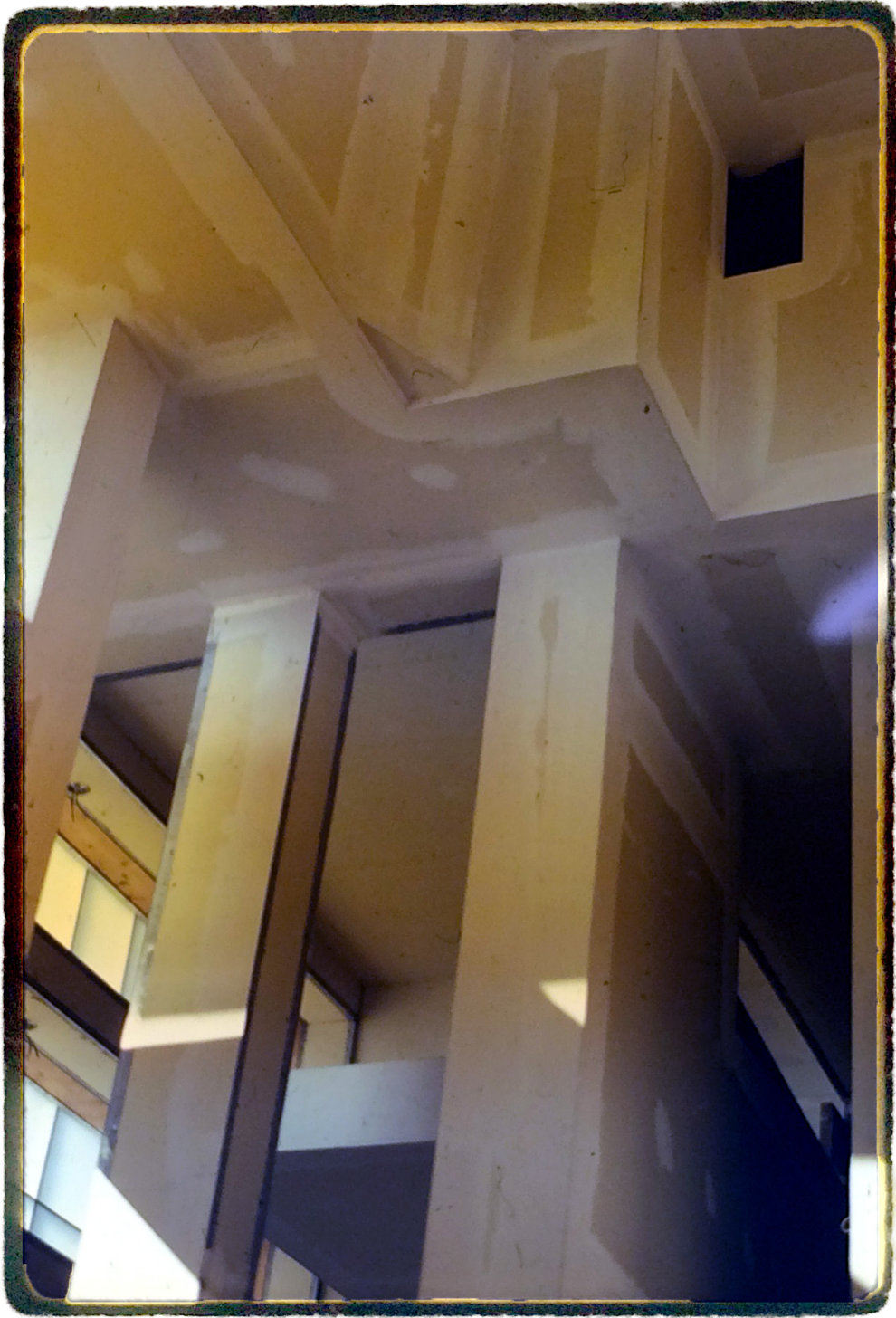
2.37 Tadas Zilius photography of Falk's house circa 1970 (drywall)
