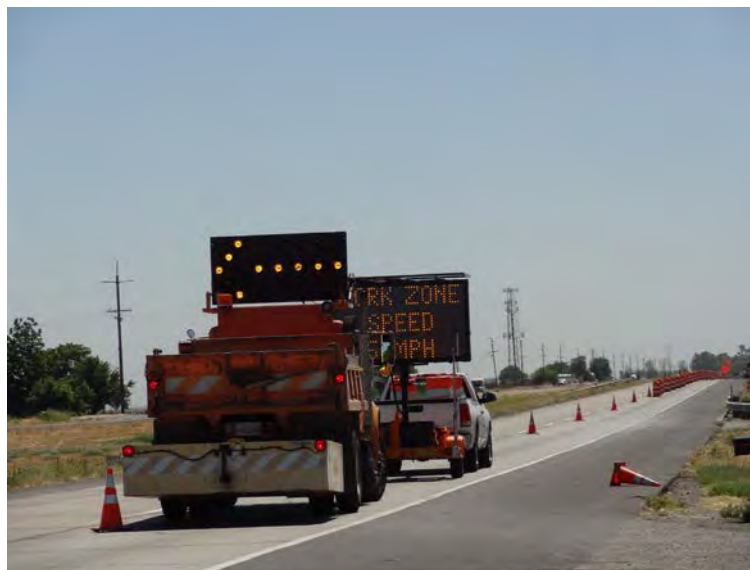
Figure 11. Equipment Setup with Assistance of Caltrans Shadow Truck
