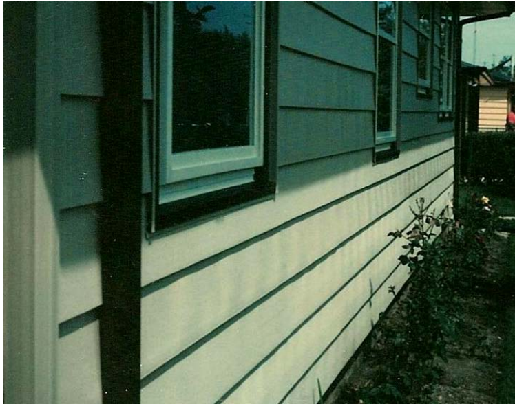
Figure 9. Vinyl siding with characteristic ripples from oil-canning (Summers 2010).
