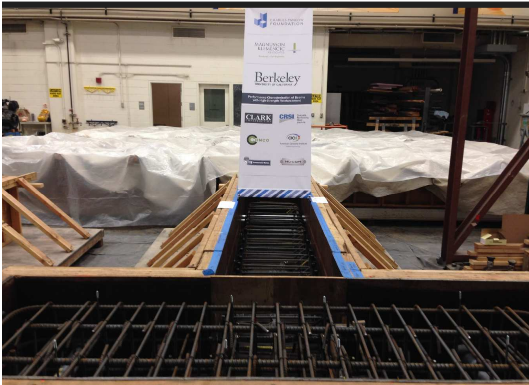
Figure A-3: Construction of Test Specimens - Reinforcement Cage
