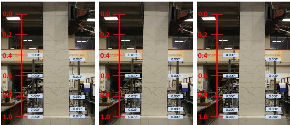
Figure C-19: Measured Crack Widths at Drift Ratio of 1.75% – Specimen SBL100
