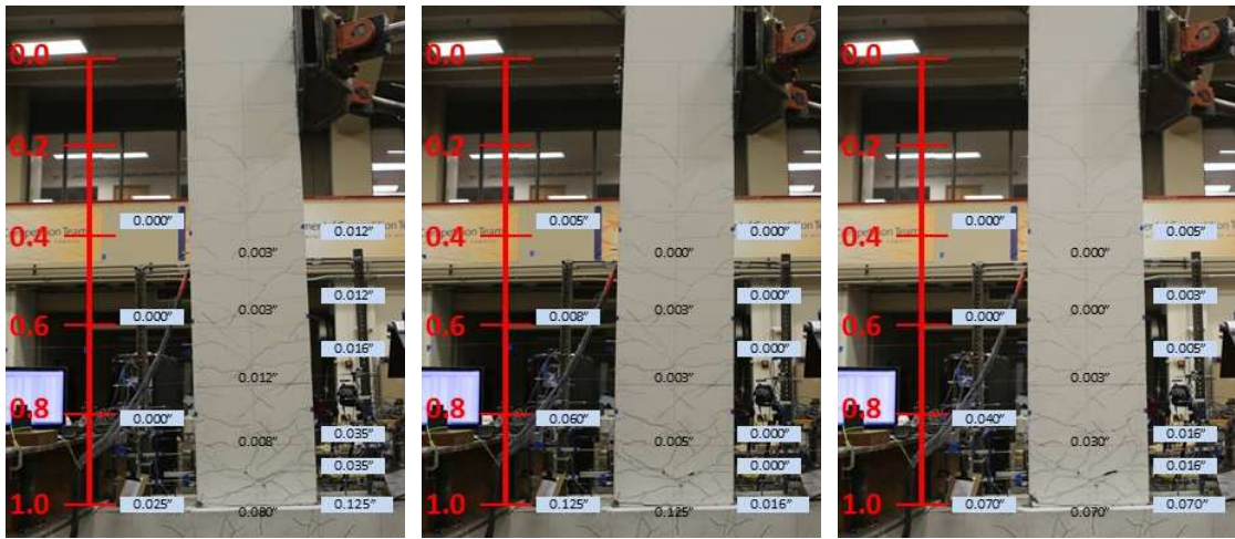
Figure C-7: Measured Crack Widths at Drift Ratio of 2.45% – Specimen SBH60
