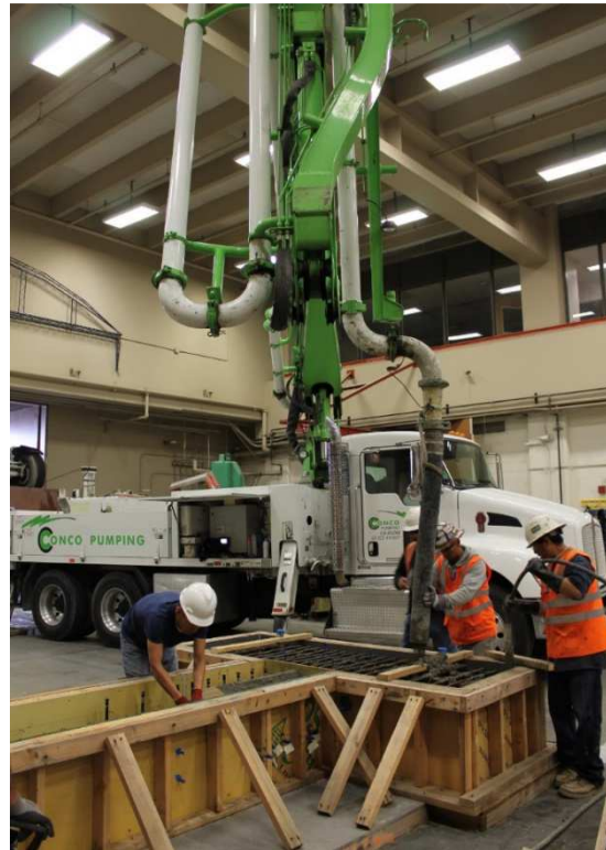
Figure A-5: Construction of Test Specimens - Concrete Casting
