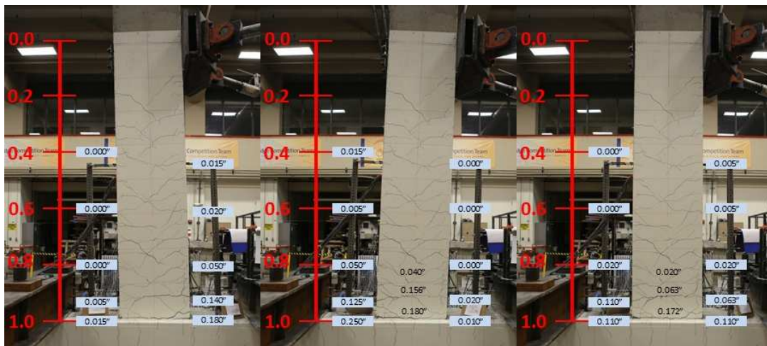
Figure C-21: Measured Crack Widths at Drift Ratio of 3.45% – Specimen SBL100
