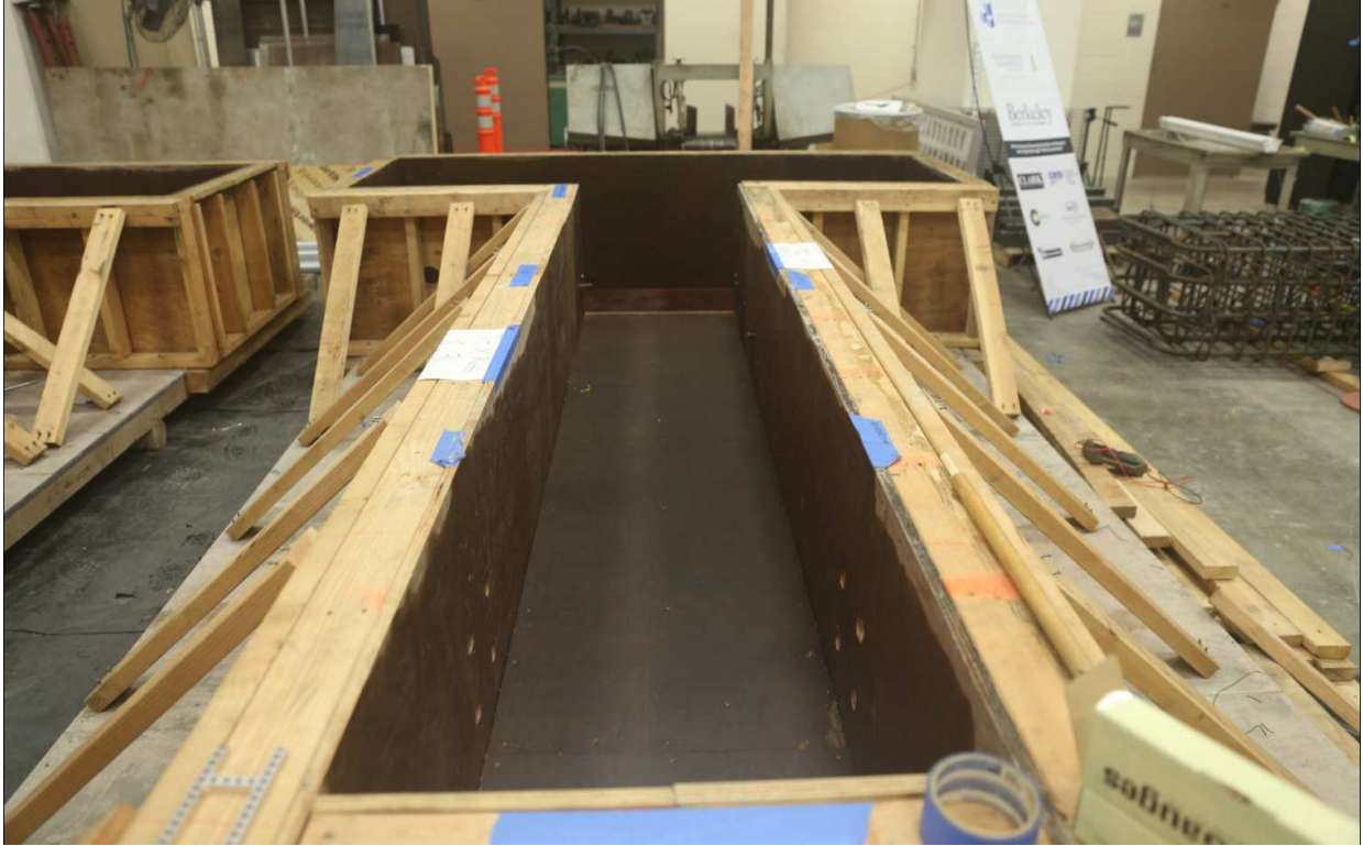
Figure A-2: Construction of Test Specimens – Formwork
