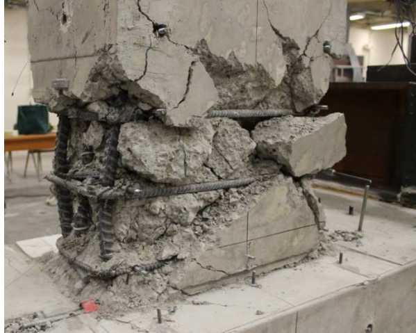
Figure 4.3.2: Failure Mechanism of SBH100 by Buckling of Longitudinal Bars Over Several Hoop Spacings
