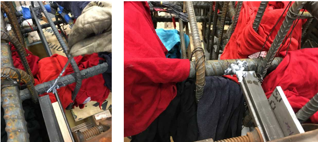
Figure A-28: Brass-Brazing Procedure - Step 2: Application of Heating Chemical
